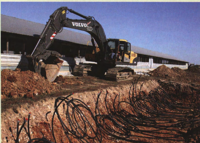
Opposite page at top, Shawn Xu, Chris Holliday and Kirby McKenzie look on as Scott Keller does some exploratory digging to see what the team will encounter when they excavate to lay horizontal heat pipes. Opposite page at bottom left, Xu examines the housings Holliday has constructed to shelter the five industrial pumps, shown, freshly unpacked, at bottom right.
