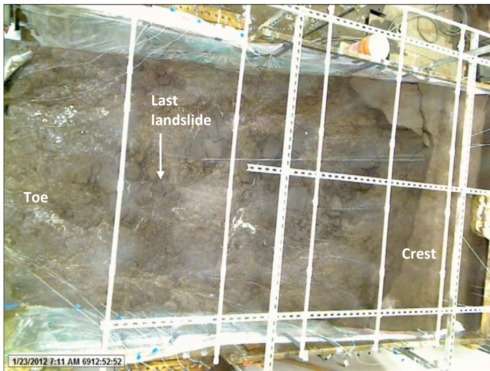
Figure 5.3 Final stage of failure, SL1 on January 23 rd after 4 days 19 hours and 16 minutes of continuous precipitation
