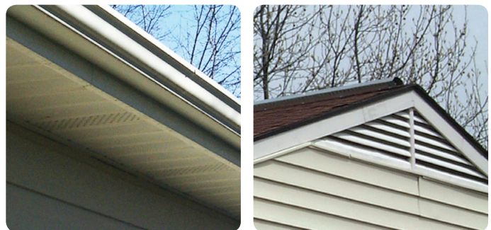
A combination of ridge and eave vents creates natural convection current, keeping your attic cool and moisture-free.
