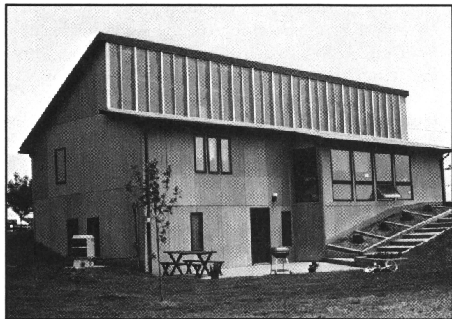
South view showing solar collector.
