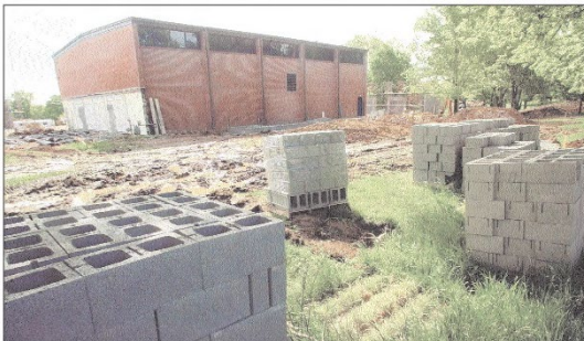
Existing Gymnasium After Demolishing the 1985 Community Center
