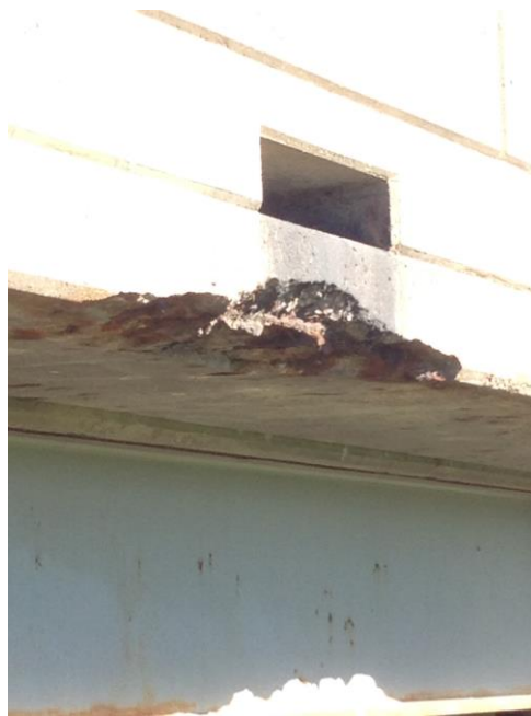
Figure 36. Close up on thickness of concrete bridge deck
