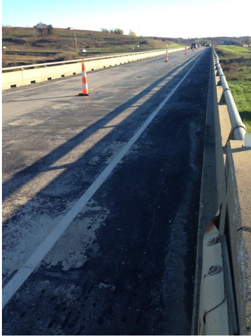
Figure 39. Bridge deck with asphalt emulsion facing east
