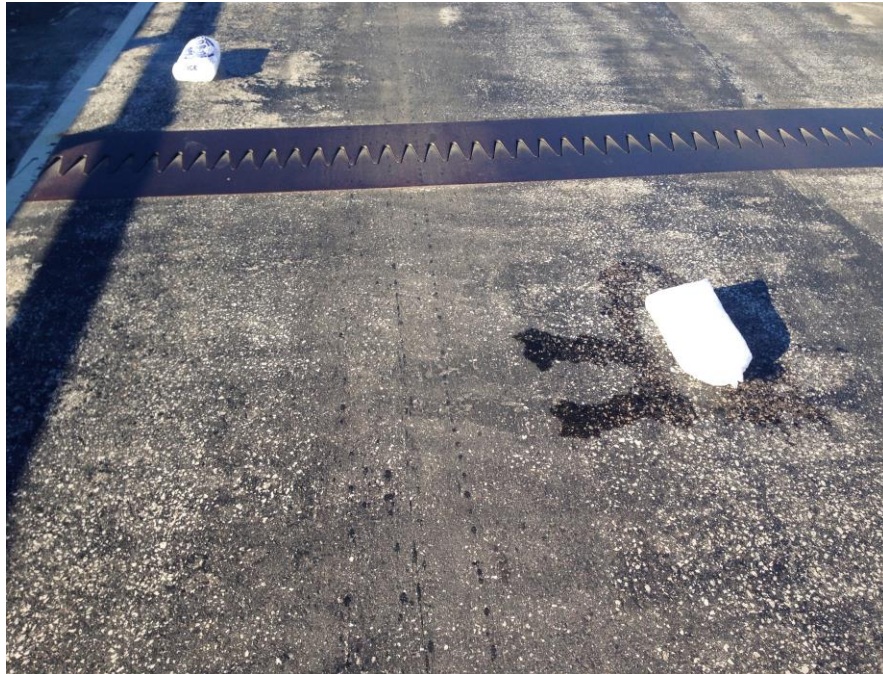
Figure 41. Expansion joint and two test sections
