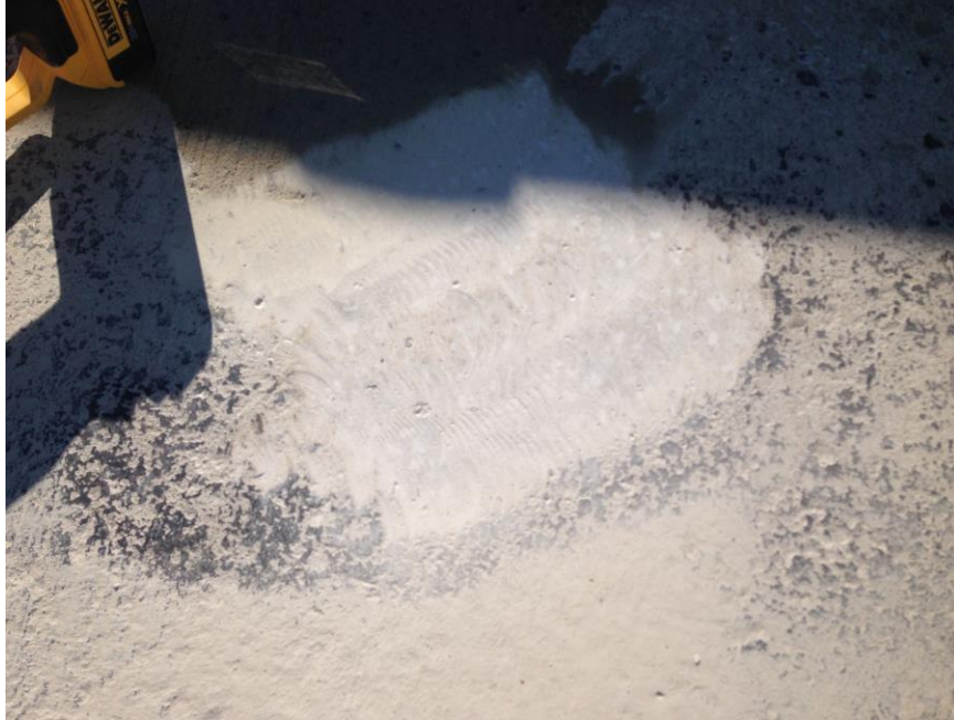
Figure 43. Ground spot where asphalt emulsion was beforehand
