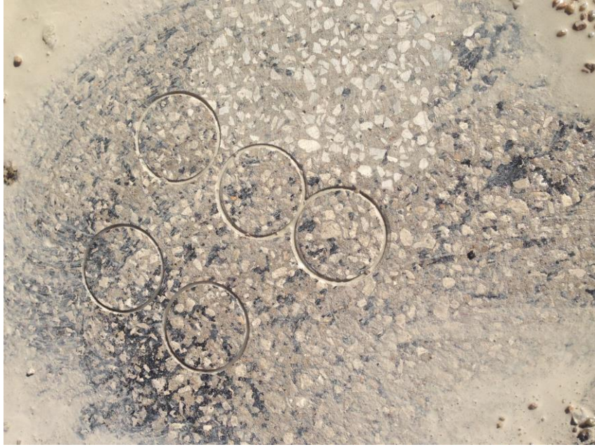
Figure 50. Five unsuccessful attempts at drilling a core of the bridge deck
