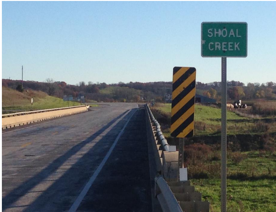
Figure 32. Shoulder view of bridge looking east
