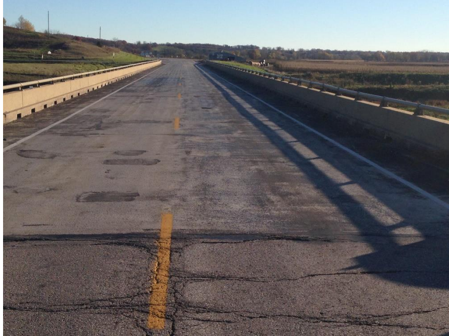
Figure 33. Center of bridge with asphalt looking east
