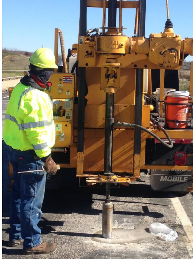
Figure 49. Drilling equipment attempting to core the concrete bridge deck
