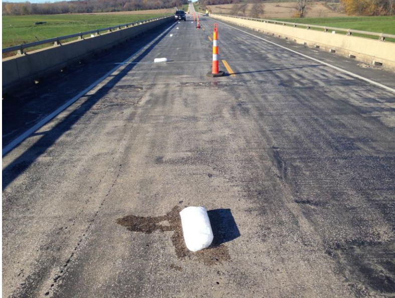
Figure 42. View of ice bags facing west on the bridge
