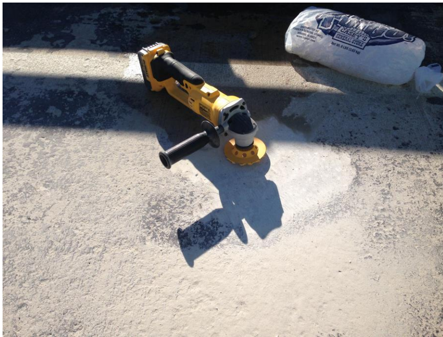
Figure 44. Angle grinder shown in a previously ground spot of pavement
