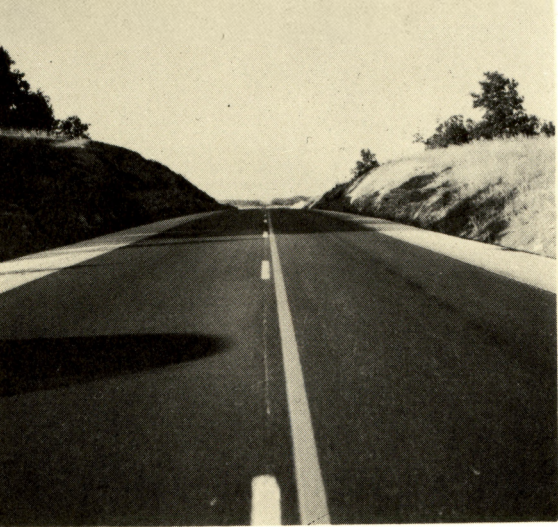
A view of new Highway 5 just North of Ava, Missouri
