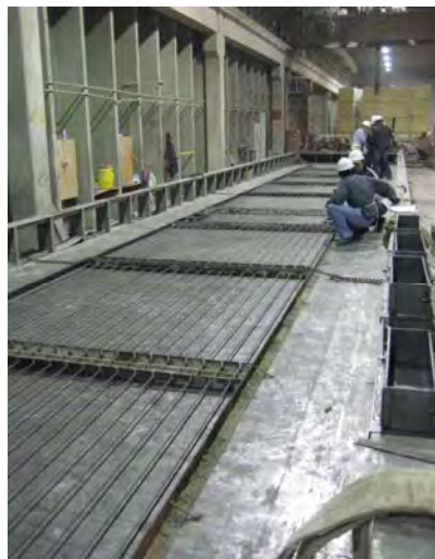
Figure C- 4 Prestressed Panel Casting Bed
