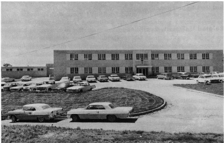
Veterinary Clinic-Hospital Building. This modern structure houses staff of clinical specialists and well-equipped surgeries and diagnostic facilities. Animals are presented for diagnosis and treatment. Students rotate through various clinical assignments for practical training and experience.
