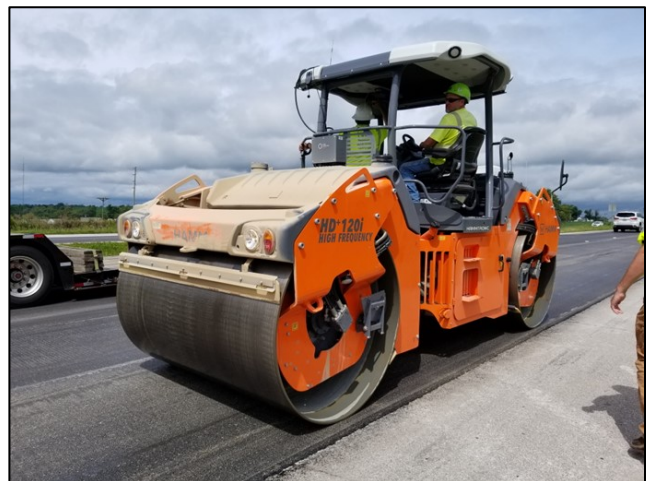
Figure 1 HAMM HCQ Intelligent Compaction System On-site (HWY 61/24 Project)
