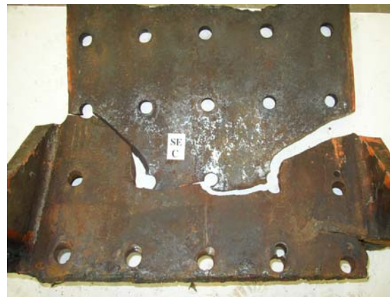
Figure 1.8 Fracture Pattern of SE Strut Web
