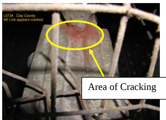
Figure 1.10 Cracking in Northeastern Strut
