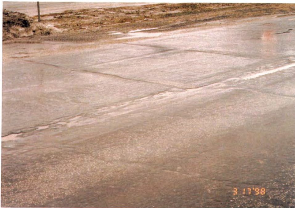
Photo #6: A slightly closer view of Photo #5. March 17, 1998; District 1, Andrew County Business Route 71
