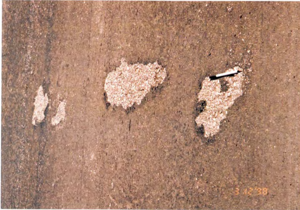
Photo #4: The inconsistent, sometimes coarse texture of the surface. March 12, 1998; District 3, Audrain County Route 22
