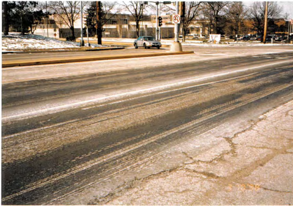
Photo #5: Coldmilling that has been performed at Litzsinger Road. March 10, 1998; District 6, St. Louis County Route 67 (Lindbergh Boulevard)
