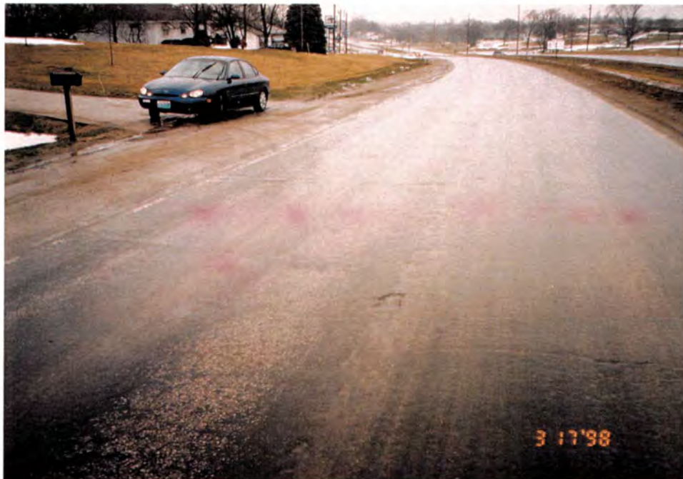
Photo #4: The driving lane (on the left) with washed sand aggregate and showing wear; the section having wet bottom boiler slag is on the right and is showing little to no wear. March 17, 1998; District 1, Andrew County Business Route 71
