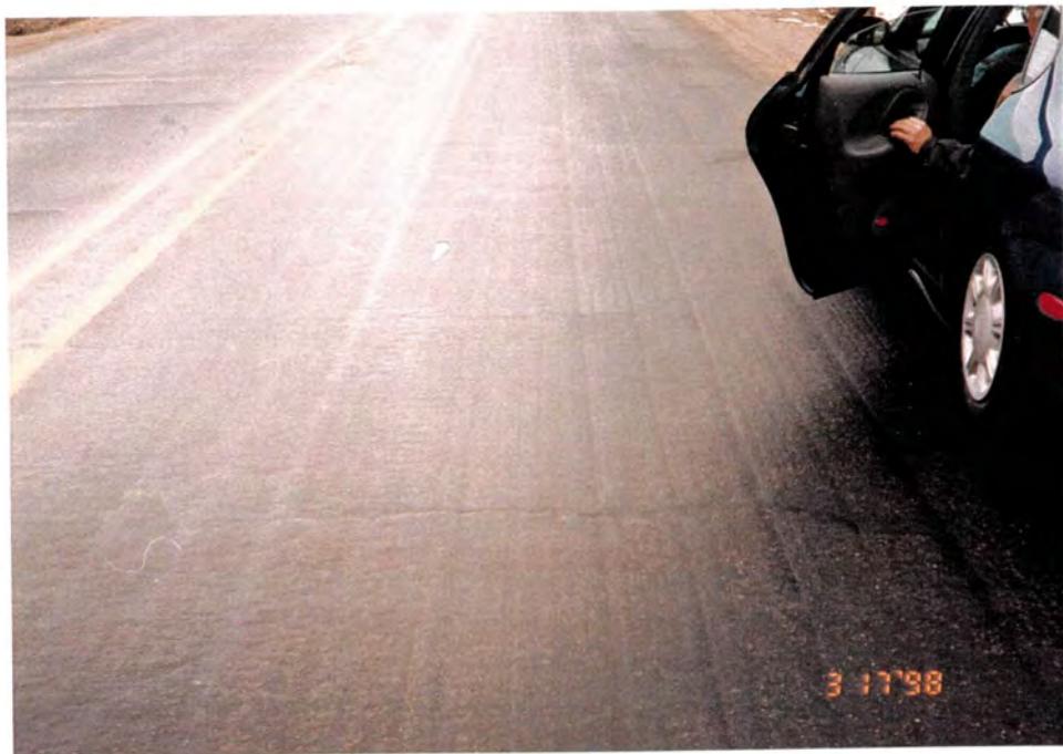
Photo #6: Another view of the surface from around 6' above. March 17, 1998; District 1, Buchanan County Route JJ
