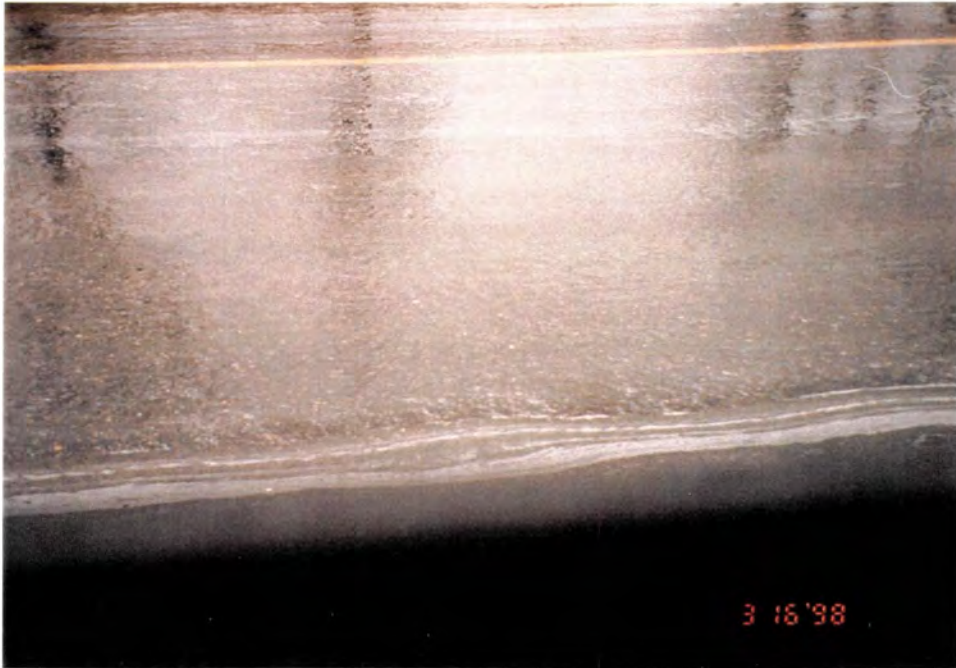
Photo #4: A concrete patch in the pavement beneath the sealant. March 16, 1998; District 2, Chariton County Route 24
