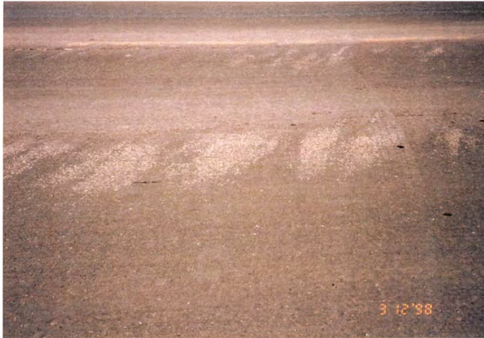
Photo #5: Snow plow damage. March 12, 1998; District 3, Audrain County Route 22
