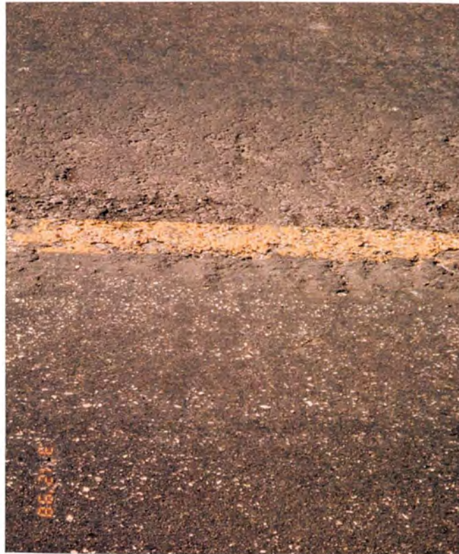
Photo #4: The inconsistent, sometimes coarse texture of the surface. March 12, 1998; District 3, Audrain County Route 22
