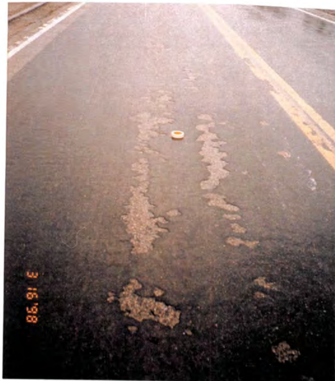
Photo #4: More wear and loss of seal. The masking tape can be seen for size reference. March 16, 1998; District 4, Lafayette County Route 24
