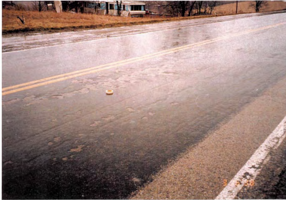
Photo #4: More wear and loss of seal. The masking tape can be seen for size reference. March 16, 1998; District 4, Lafayette County Route 24
