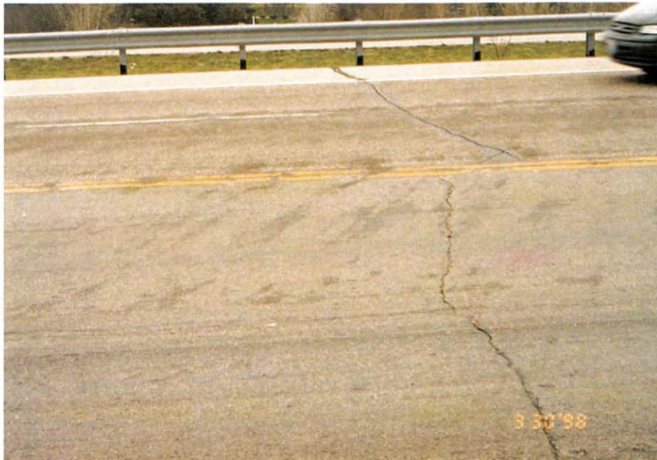
Photo #2: A view of the seal lane (closest) and the unsealed lane. March 30, 1998; District 5, Cole County Business Route 50 (Missouri Boulevard)
