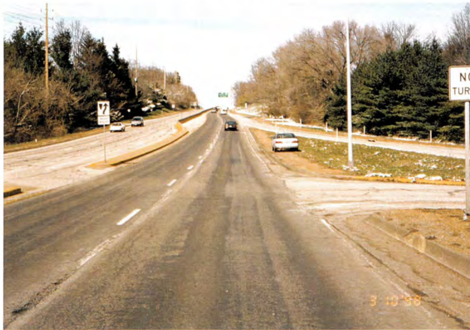
Photo #1: View up the hill leading to the Frontenac city limits. The seal is almost gone in the wheelpaths. March 10, 1998; District 6, St. Louis County Route 67 (Lindbergh Boulevard)
