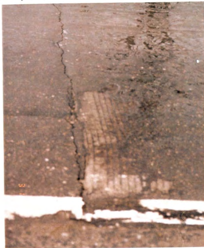
Photo #4: A concrete patch in the pavement beneath the sealant. March 16, 1998; District 2, Chariton County Route 24
