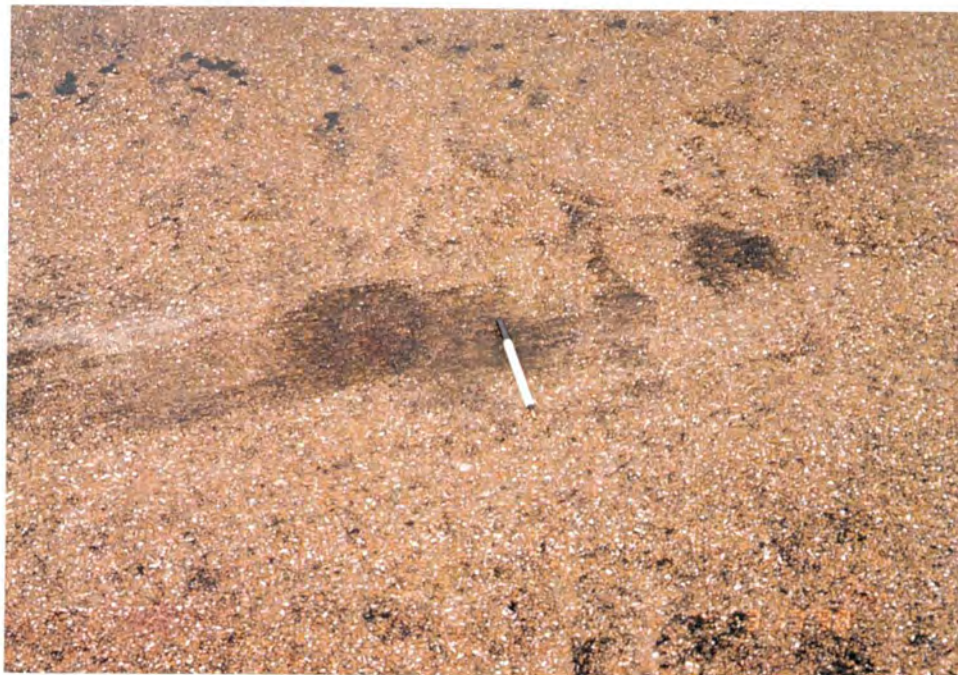
Photo #2: A close-up view of the surface, showing a mild snowplow scar. An inkpen is shown for size reference. March 17, 1998; District 4, Henry County Route H
