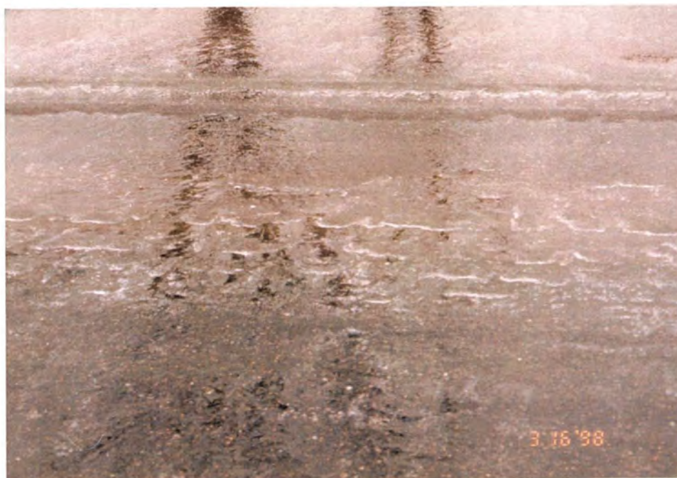
Photo #1: Sheet flow on the driving surface. March 16, 1998; District 2, Chariton County Route 24
