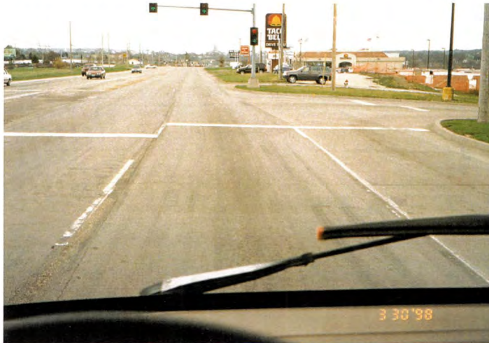
Photo #1: A view of the surface at the turnoff to Wal-Mart. March 30, 1998; District 5, Cole County Business Route 50 (Missouri Boulevard)
