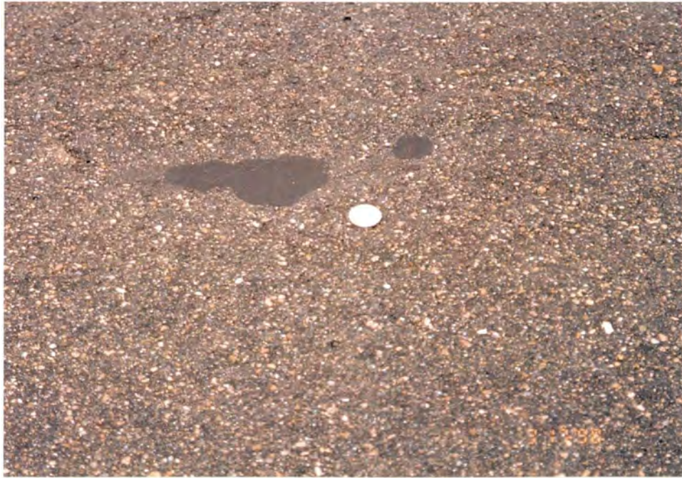
Photo #3: Splotches of emulsion on the surface. A quarter is shown for size reference. March 17, 1998; District 4, Henry County Route 52
