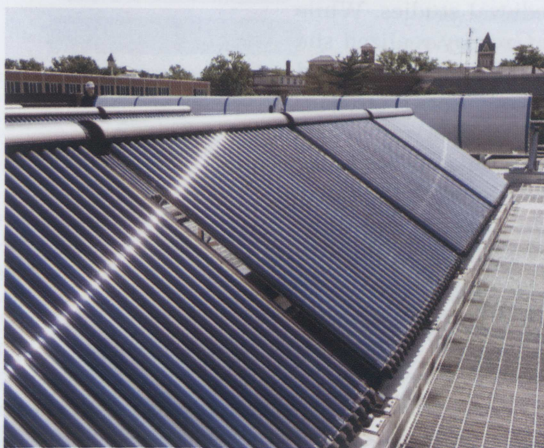
↑ MU's power plant installed a solar rooftop thermal system that reduces coal usage and MU's carbon footprint.
