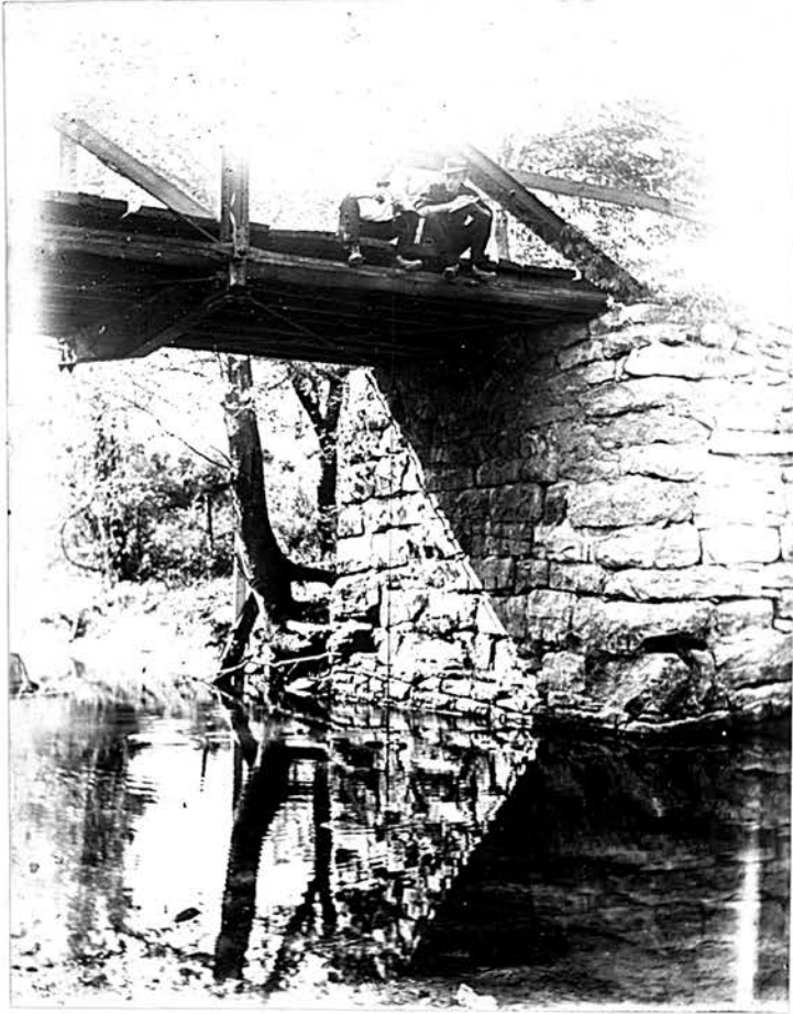
Method of taking High Water Observations
