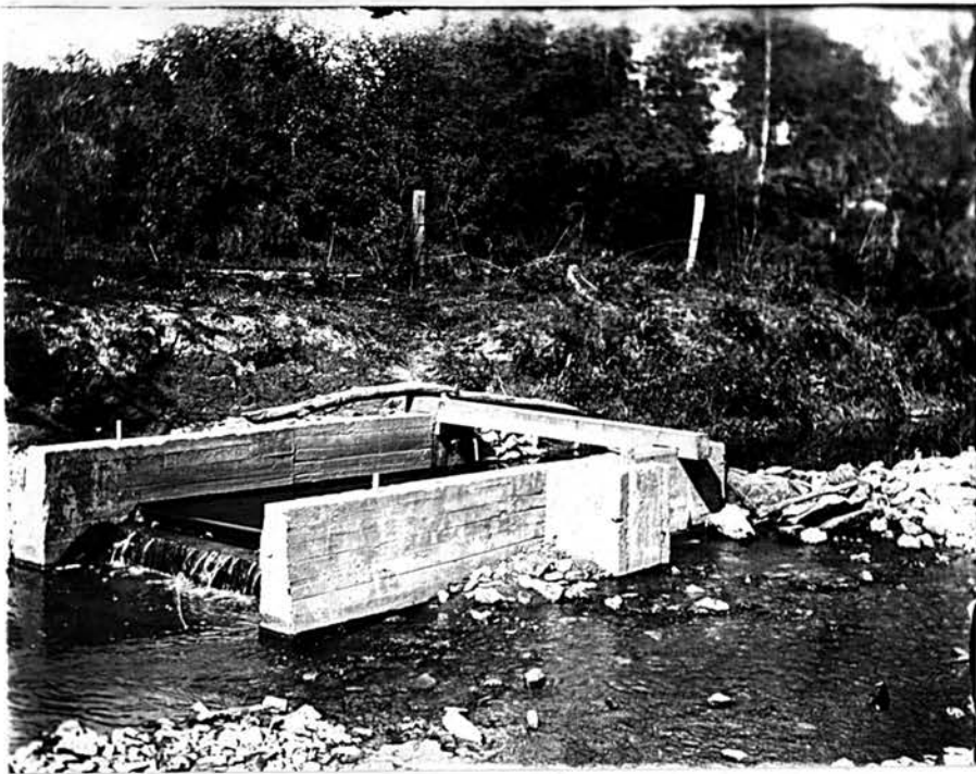
The Weir Showing results of failure of dam.
