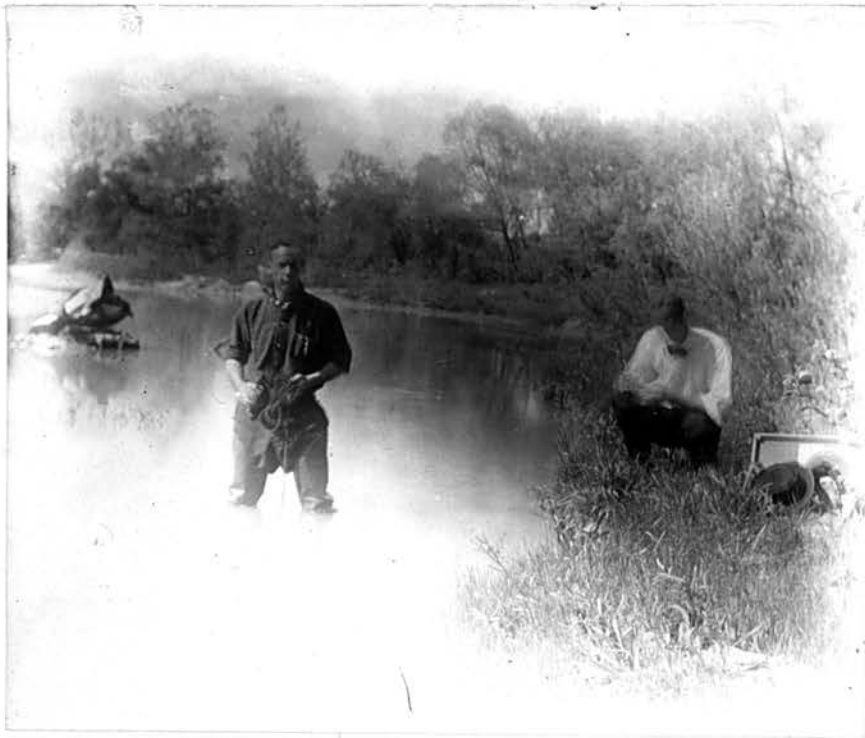
Wading Section with Price Meter
