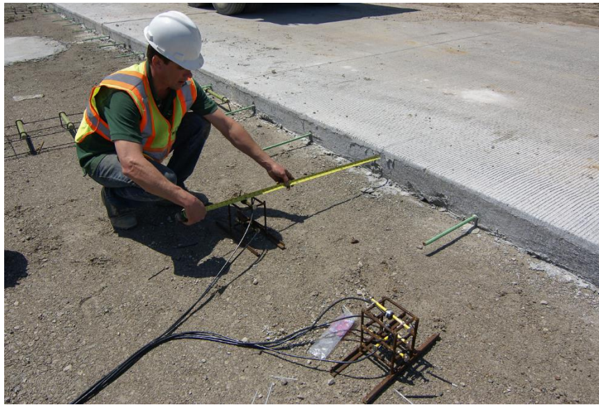
Figure 6-1. Photos of the location of the sensors
