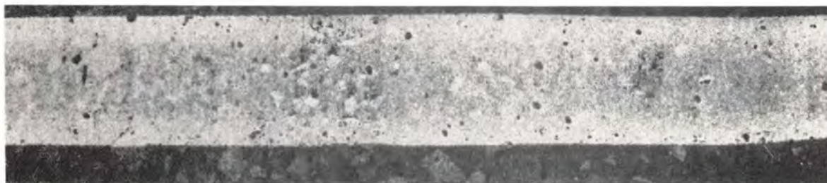
Figure 9c - Photographic Record of High Heat Paint Type "G", White, on Concrete Pavement
