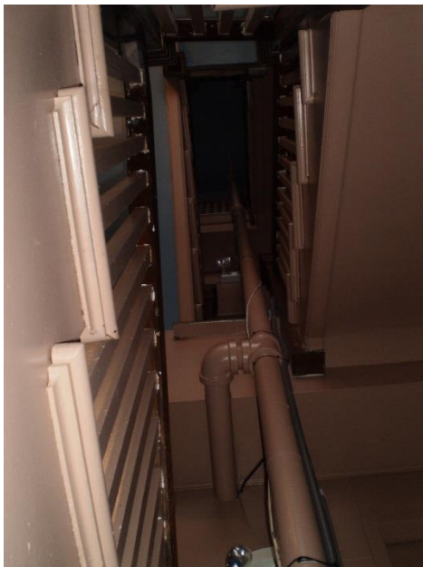
Figure 23. Lakeshores RCF stairwell Elevator
