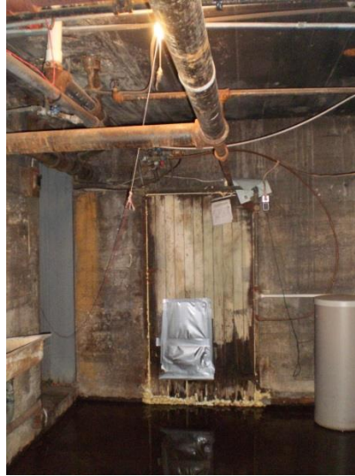
Figures 26. Lakeshores RCF Opening in Basement for Coal
