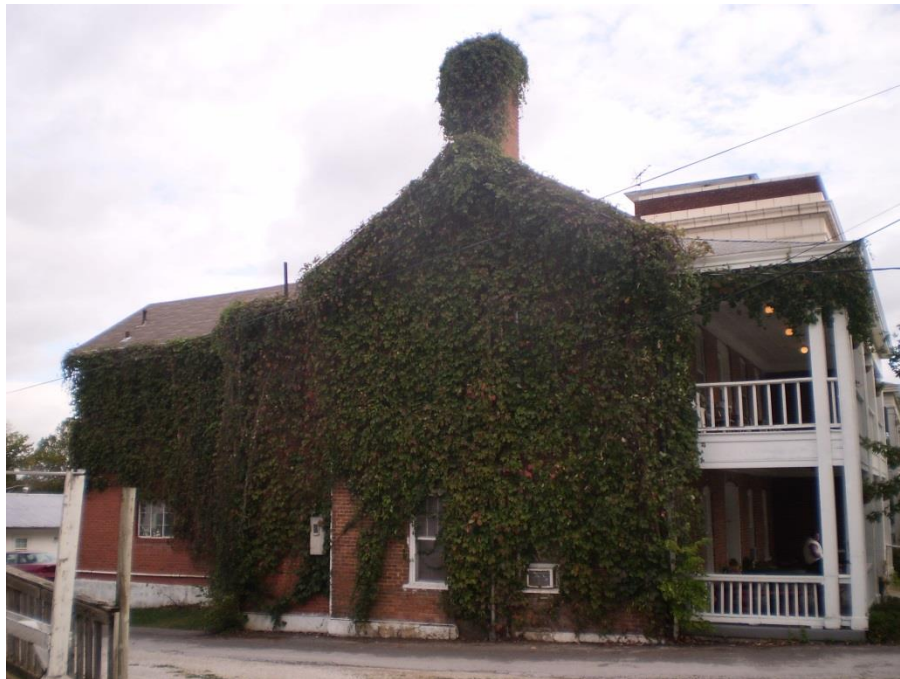
Figure 10. Lakeshores Residential Care Facility North side
