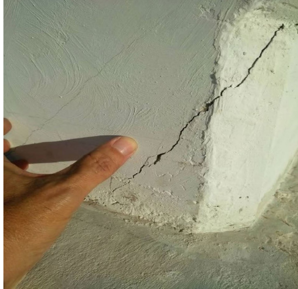
Figure 1-3 Cracking of truss member 11 after bridge placement [1]
