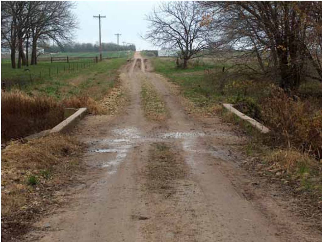
View across the bridge to the east
