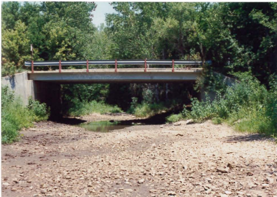
Sideview Looking North
