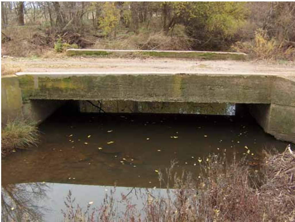
Profile view of the bridge to the south
