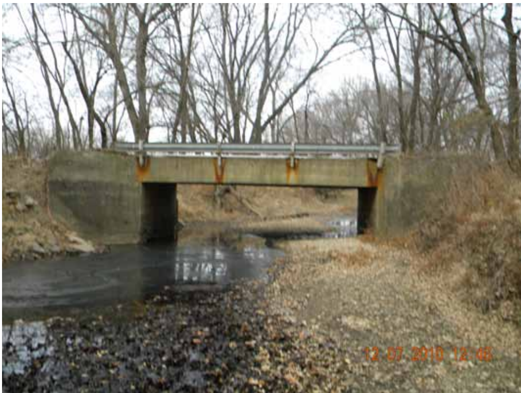
Profile view of the bridge to the north
