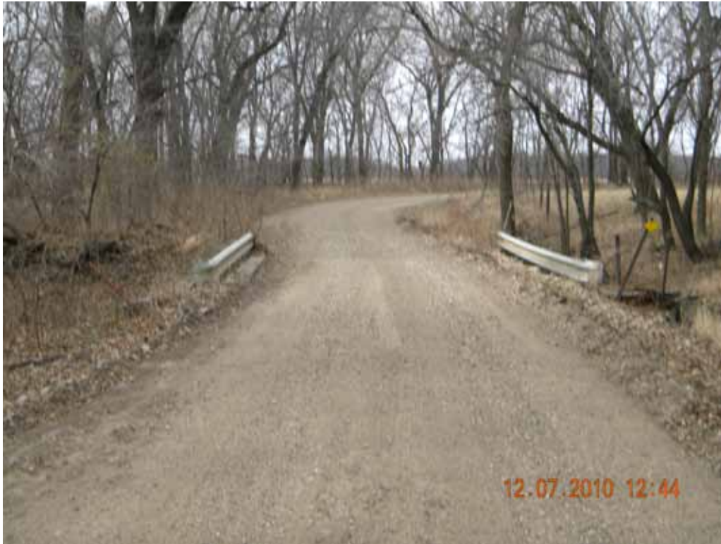
View across the bridge to the west
