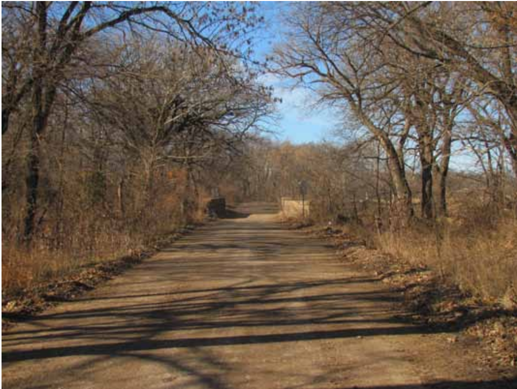
View across the bridge to the west
