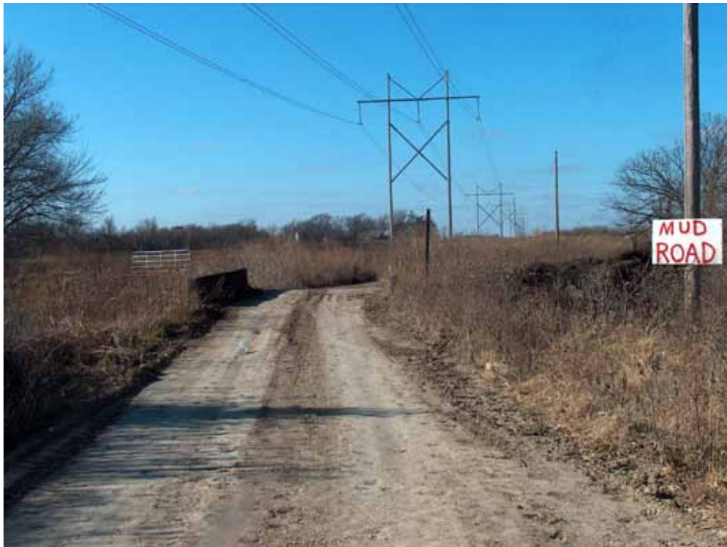
View across the bridge to the west
