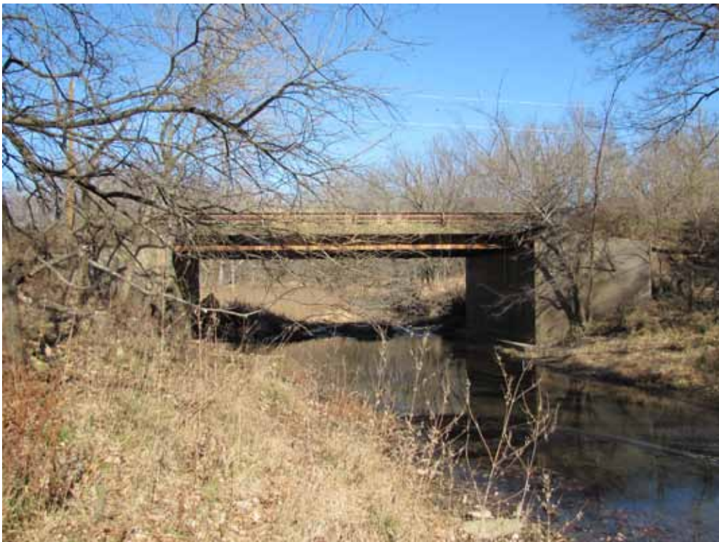
Profile of the bridge to the north
