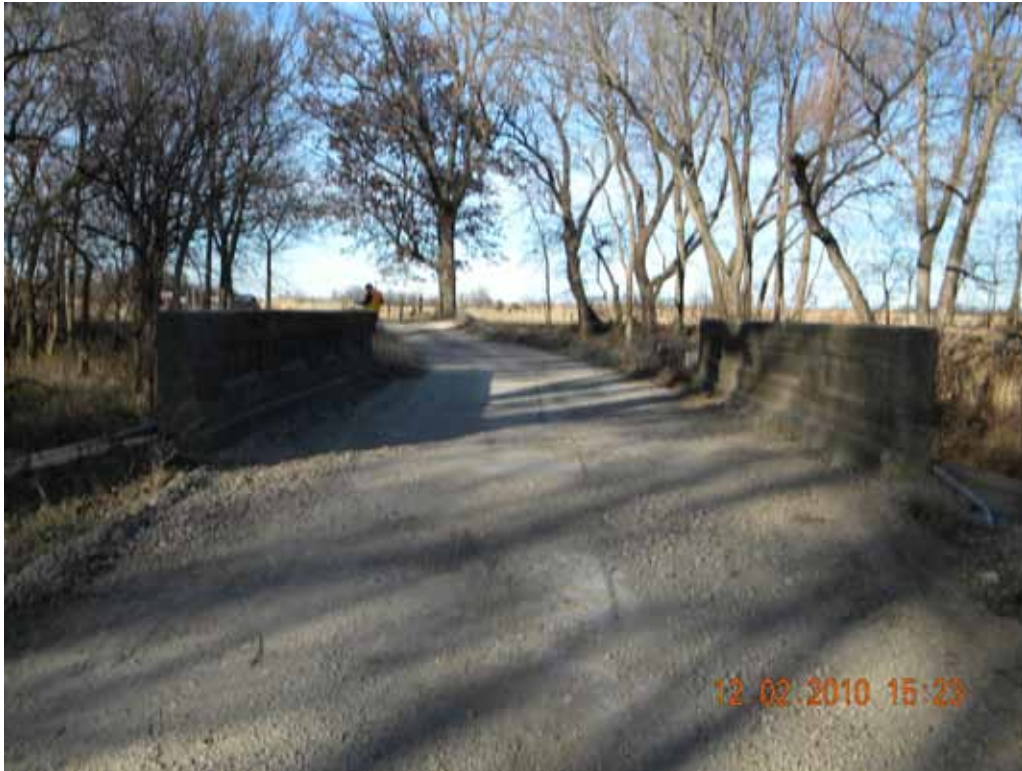
View across the bridge to the north
