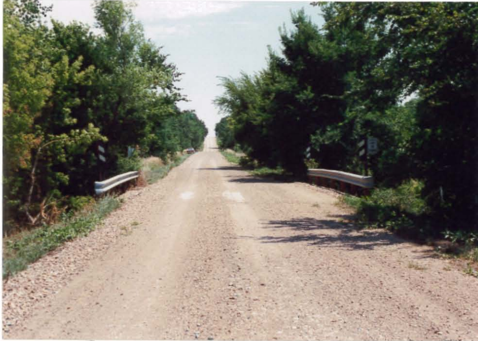
Roadway Looking East
