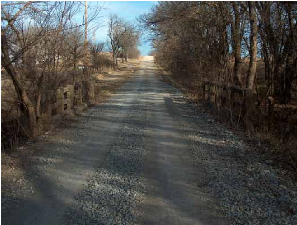
View across the bridge to the east
