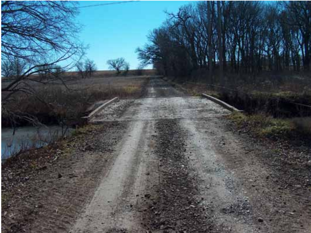
View across the bridge to the south
