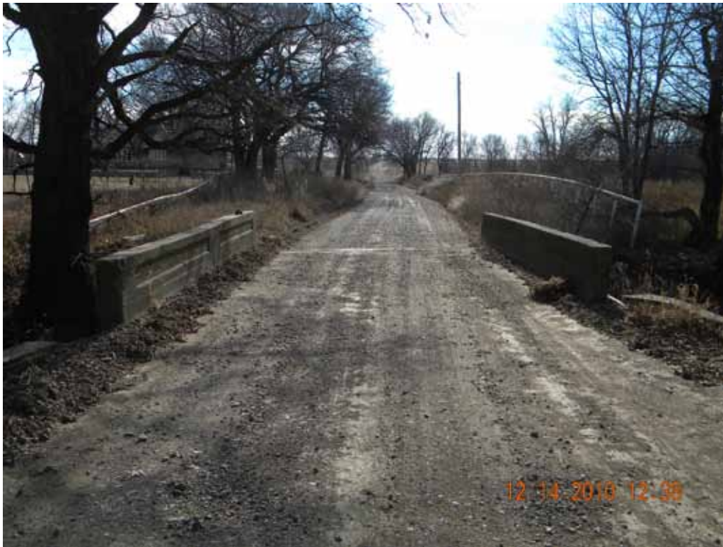
View across the bridge to the south
