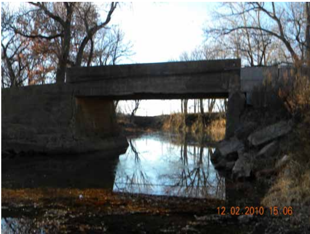
Profile view of the bridge to the west
