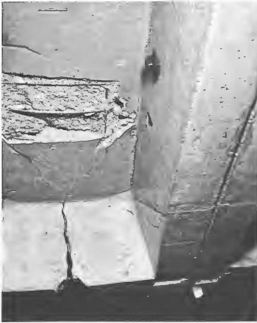
Figure 25. Diaphragm failure.
