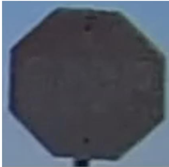
Figure 11. Faded Stop Sign
