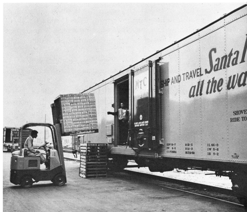
Frozen orange juice being loaded in mechanical refrigerator car. —Santa Fe Railway photo
