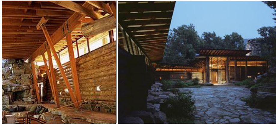
Figure 32. Two views of Bohlin Cywinski Jackson's Ledge House, Maryland.
