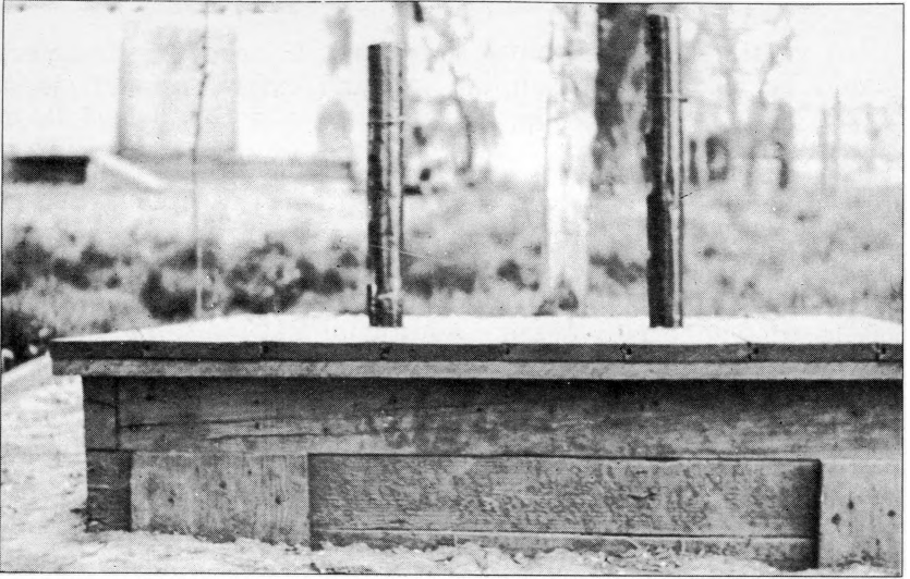
Fig. 1.—Inexpensive hole-in-the-ground egg cooler.
