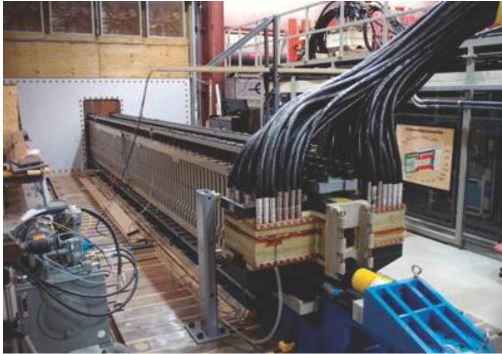
Figure 1. 2: The capacitor bank that powers the Navy's Electromagnetic Railgun (EMRG) [3]
