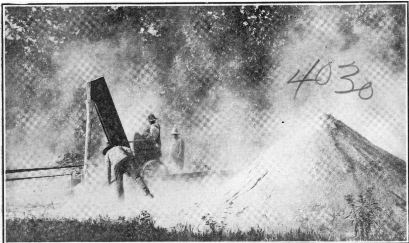
FIG. 8.—Twenty-five limestone pulverizers were introduced in 1920
