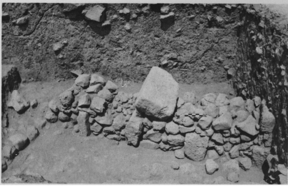
Trench in the eastern area with wall showing re-use of ashlar blocks.
