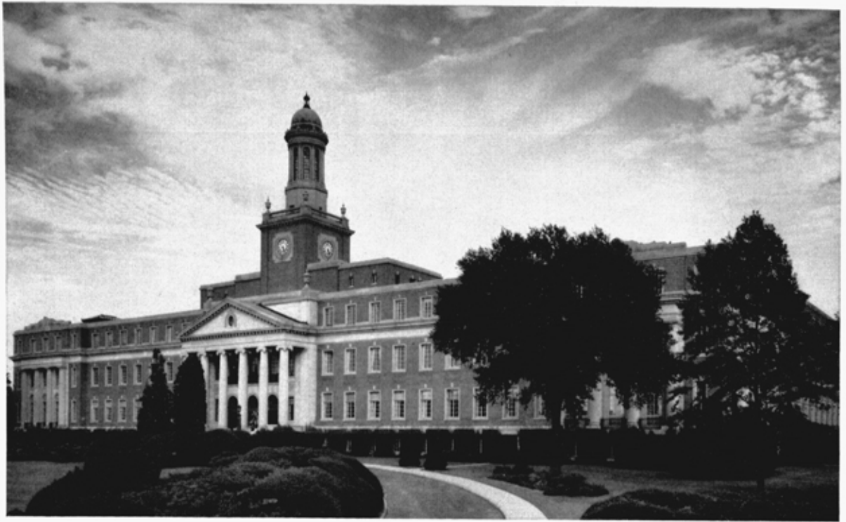
Massachusetts Mutual Home Office
