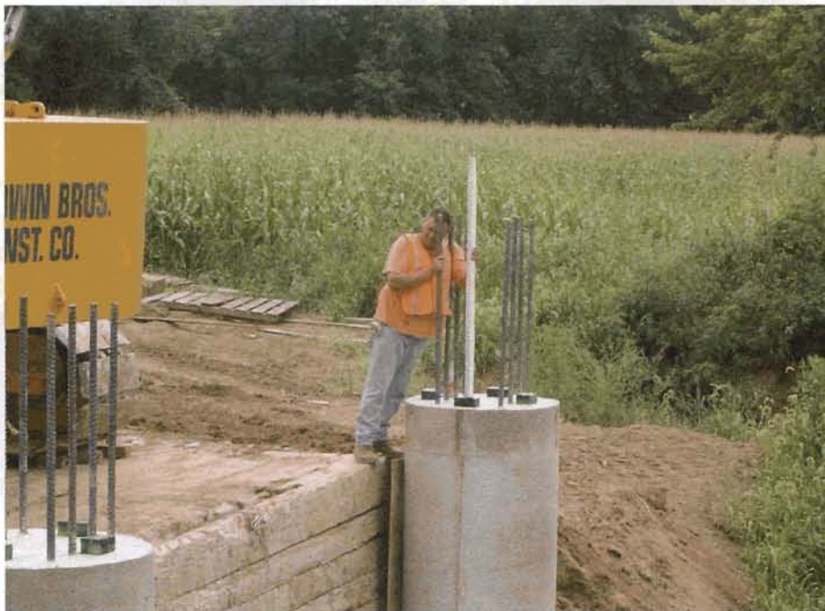
Figure 5.2 Checking Elevations of Shim Plates
