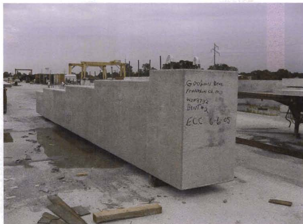
Figure 4.5 Finished Beam Cap
