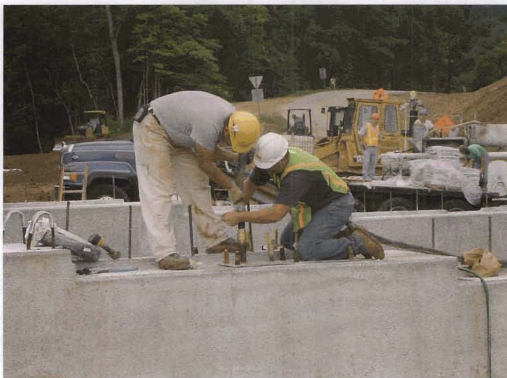
Figure 6.4 Attaching Hose to Inlet Valve in Plate
