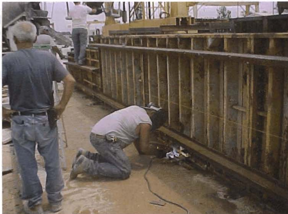
Figure 4.4 Reinforcing Formwork
