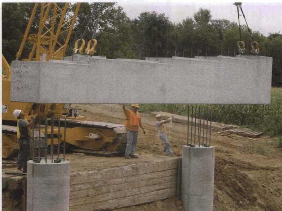
Figure 5.3 Setting Beam Cap at Bent No. 3
