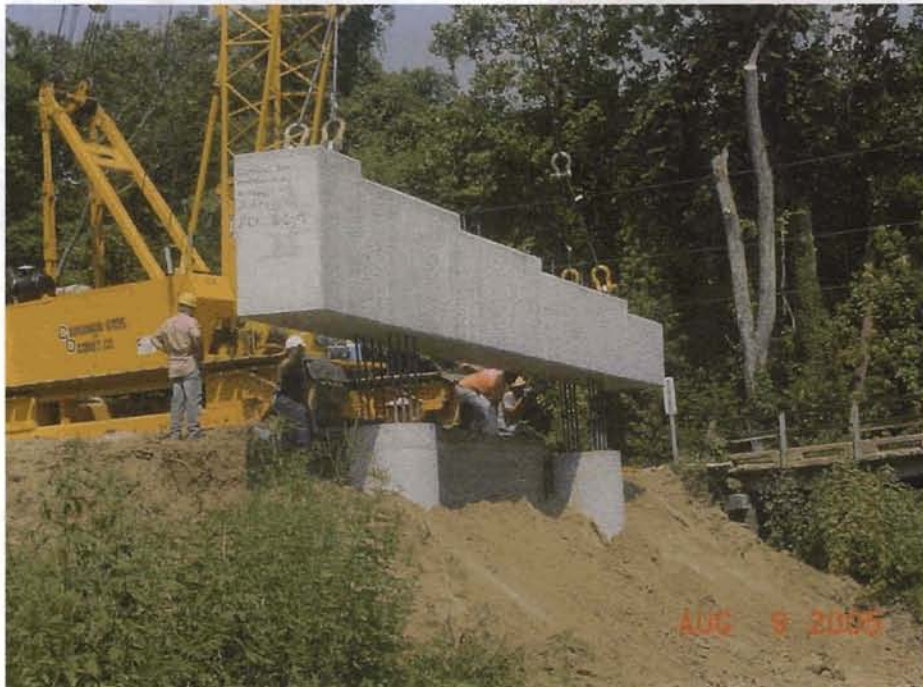
Figure 5.5 Setting Beam Cap at Bent No. 2
