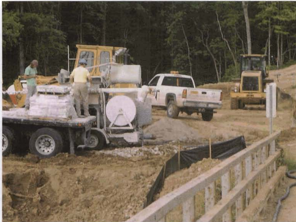
Figure 6.3 Grout Mixer and Hose to Pump Grout to Beam Cap
