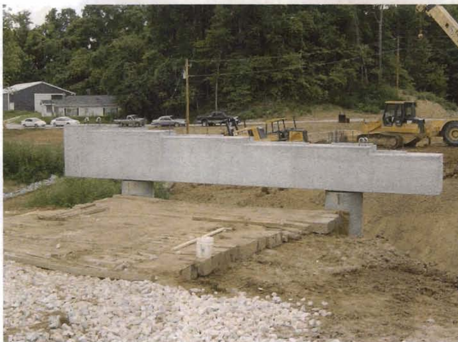
Figure 5.6 Beam Cap in Place after Setting
