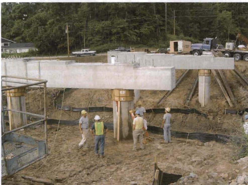
Figure 6.2 Checking if Forms are Watertight
