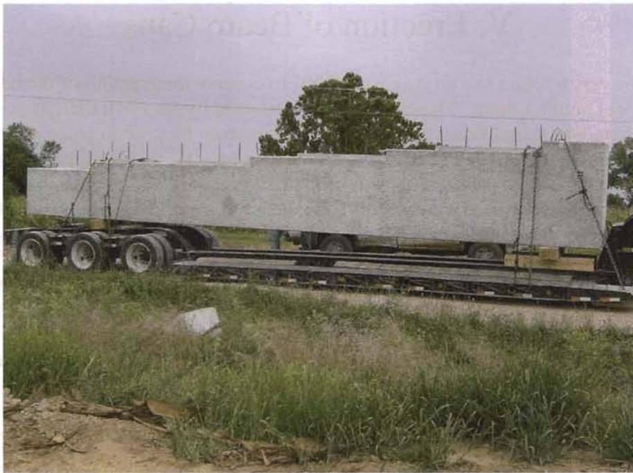
Figure 5.1 Beam Cap Delivered by Tractor Trailer
