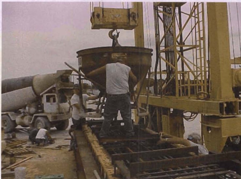
Figure 4.3 Placing Concrete by Crane and Bucket
