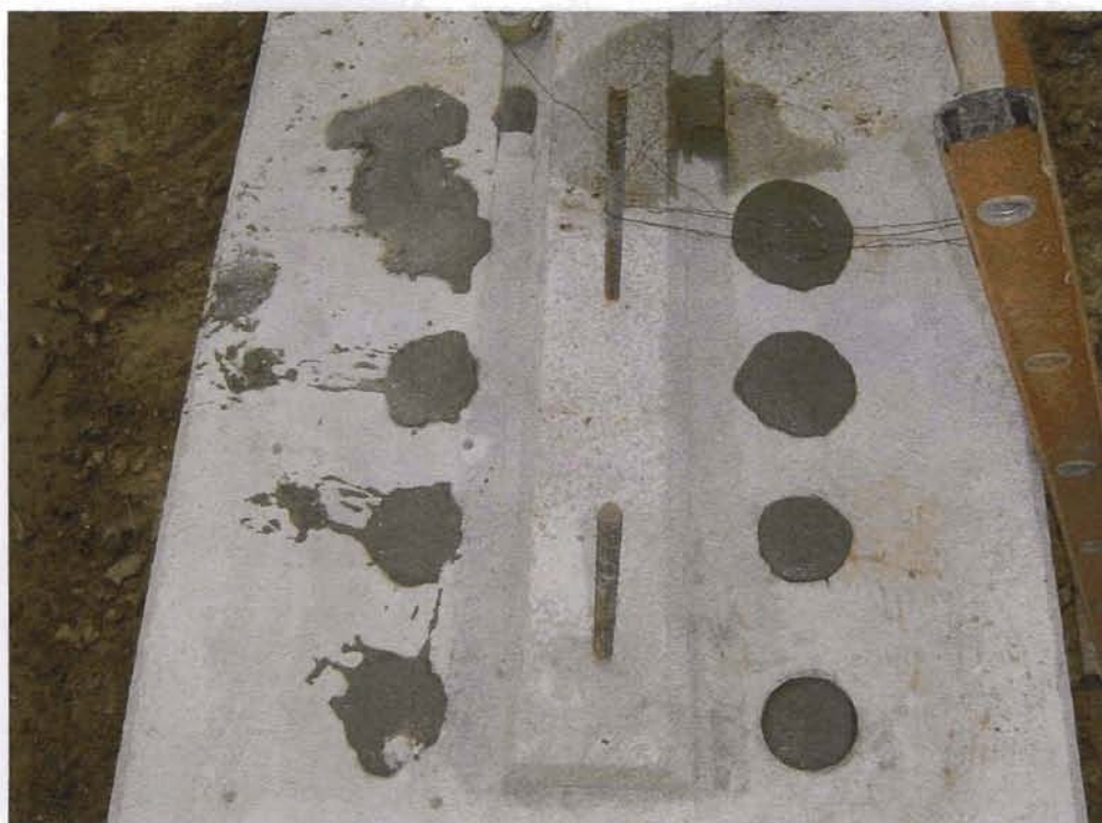
Figure 6.6 Filled Grout Tubes after Grouting Process
