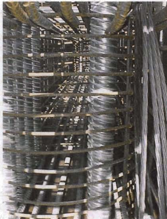
Figure 4.1 Rebar Cage and Grout Tubes
