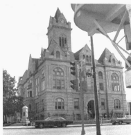
Cole County Courthouse, Jefferson City
