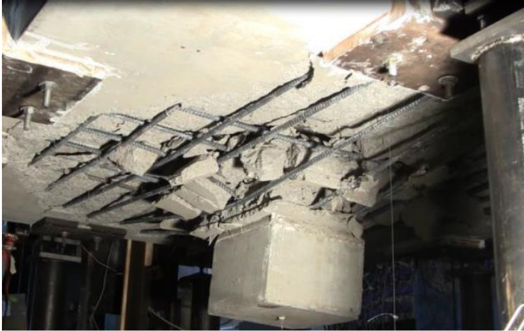
Figure 4.4.2.3 – Underside of 1.0% static test at the conclusion of testing
