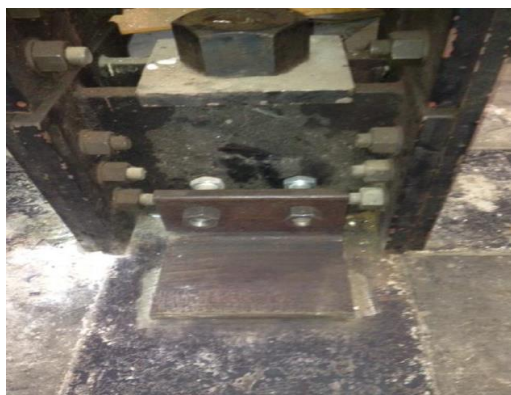
Figure 3.4.7 – Angle stops welded at the base of each vertical column
