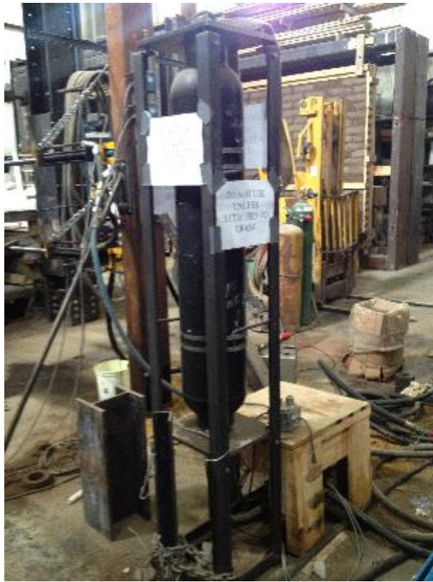
Figure 3.4.10 – Hydraulic tank used to power ram
