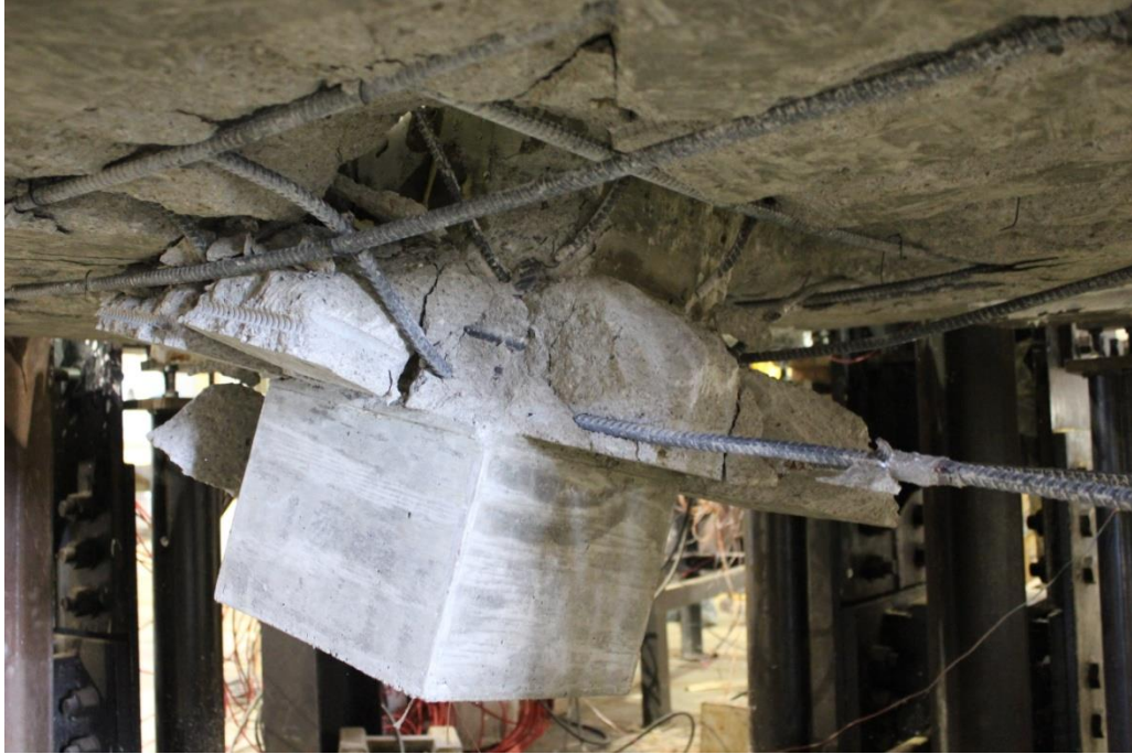
Figure 4.1.7 – Dynamic test 1 after failure of the connection
