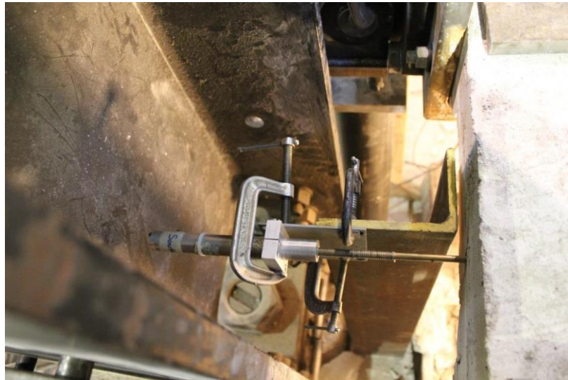
Figure 3.5.5 – Picture from above slab showing LVDT against outer face of slab
