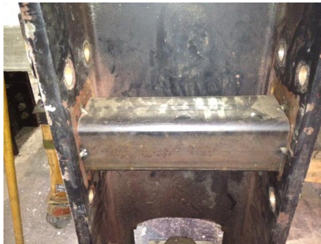
Figure 3.4.8 – Compression brace welded to support columns
