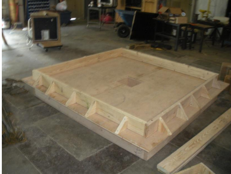
Figure 3.3.1 – Completed isolated slab formwork without top column form in place
