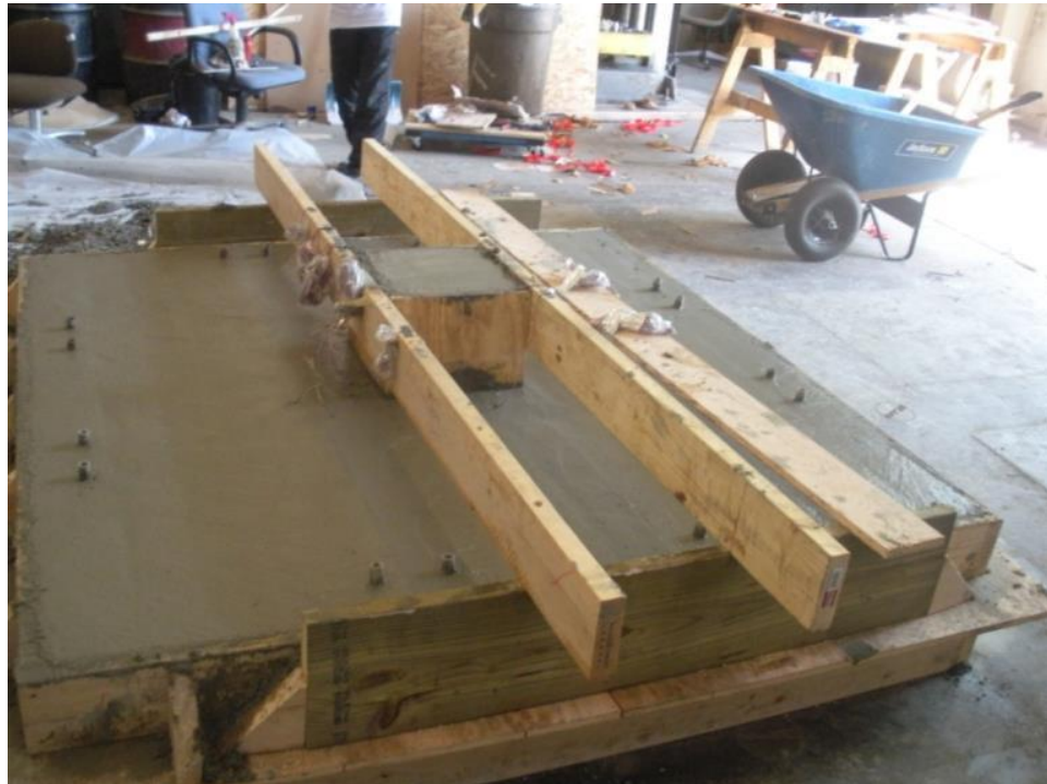
Figure 3.3.4 – Slab after pouring and surface finishing was complete
