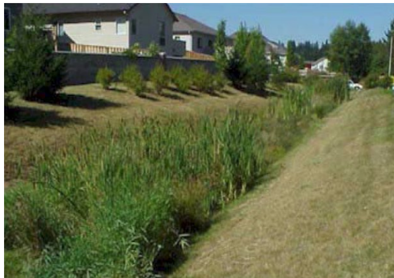
Figure 1.6: Example of Vegetated Swale (Pennsylvania Department of Environmental Protection, 2007)
