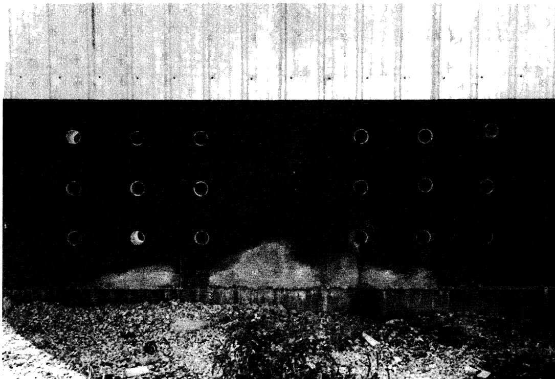
Air enters the compost bins through holes in the compost bin walls.
