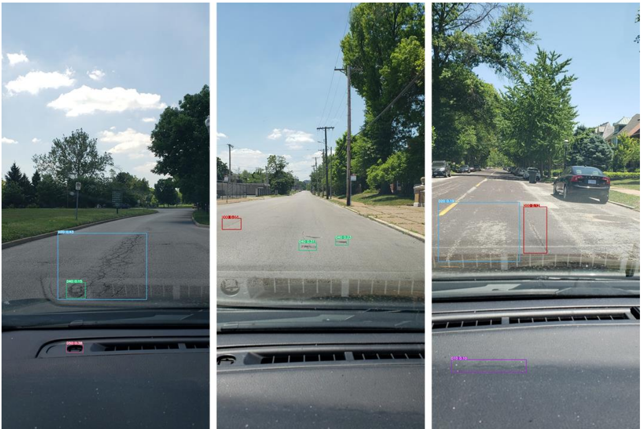
Figure 2.16: Pavement distresses detected from video data
