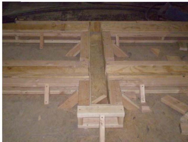
Figure 3.5.5: Construction of formwork
