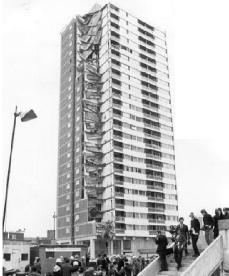
Figure 2.1.1: Ronan Point Tower after collapse (Nair, 2004)
