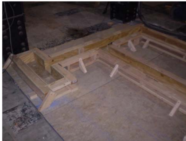
Figure 3.5.2: Construction of formwork
