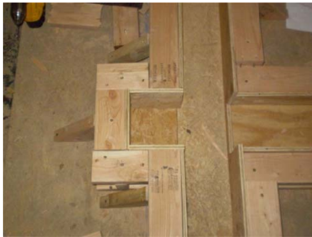
Figure 3.5.4: Construction of formwork
