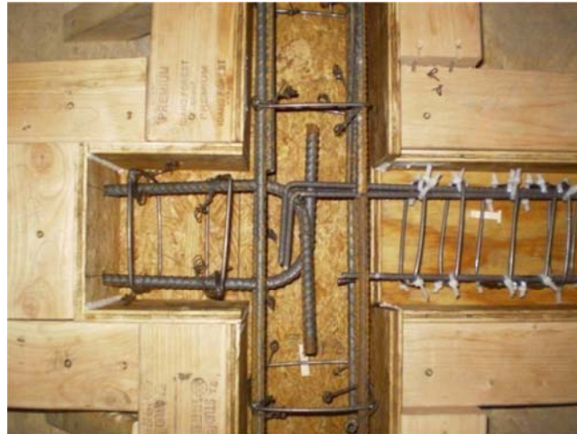
Figure 3.5.15: Hooked #4 end-threaded bars
