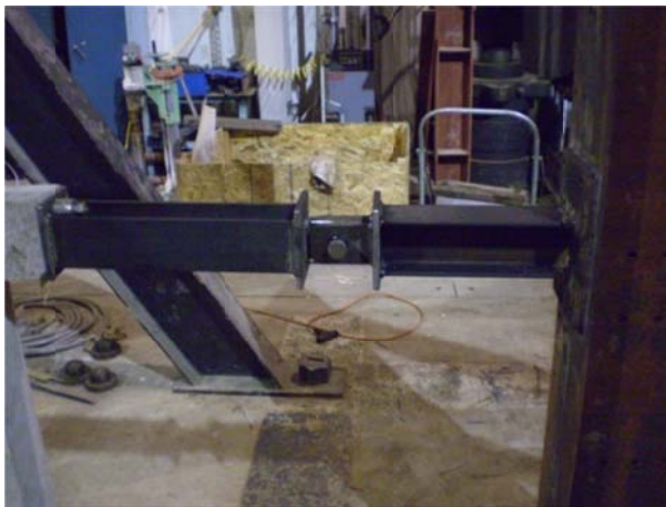
Figure 3.6.6: Reaction frame tied into the concrete frame
