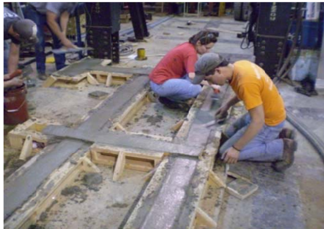
Figure 3.5.21: Smoothing out the concrete
