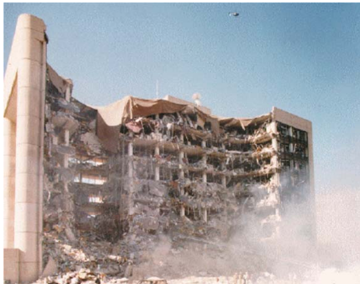
Figure 2.1.2: Murrah Building after explosion (Crawford, 2002)
