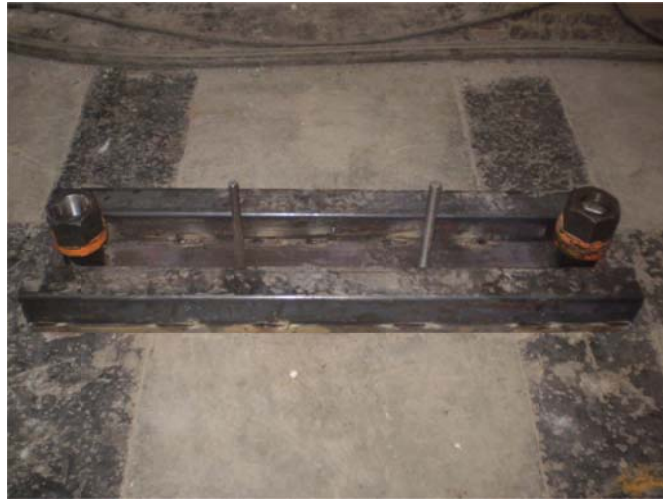
Figure 3.6.8: Anchor for the pedestal
