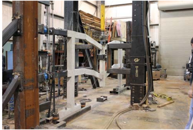
Figure 4.1.2: Discontinuous frame forming cracks
