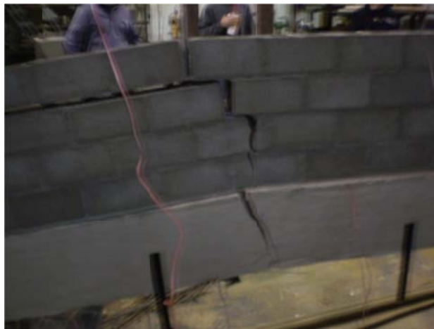
Figure 4.3.10: Crack propagates through beam
