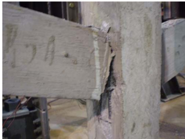
Figure 4.1.8: Formation of cracks at the center column
