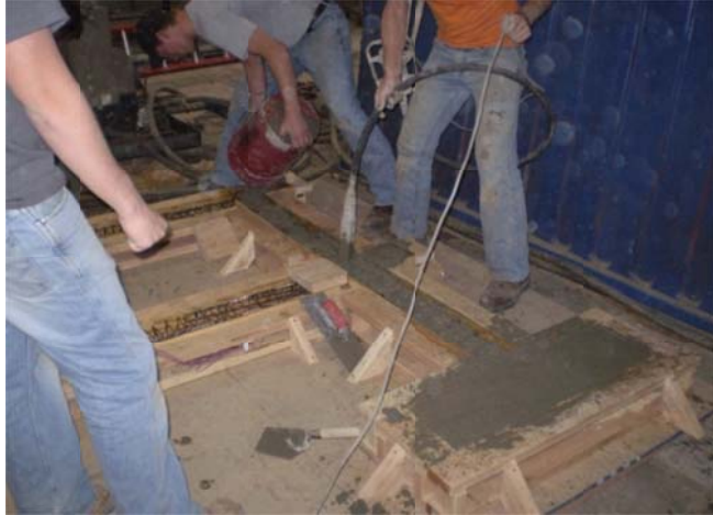
Figure 3.5.20: Pouring and vibrating concrete
