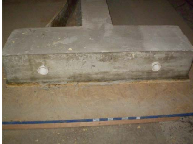
Figure 3.5.25: PCP pipes in pedestals
