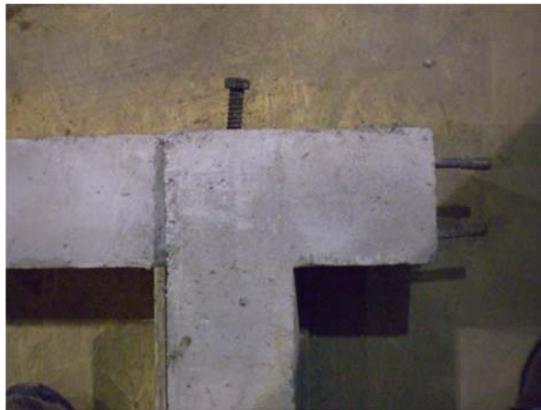
Figure 3.5.24: Lifting insert and end-threaded bars
