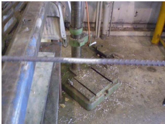
Figure 3.5.12: Bars grinded and scrubbed clean
