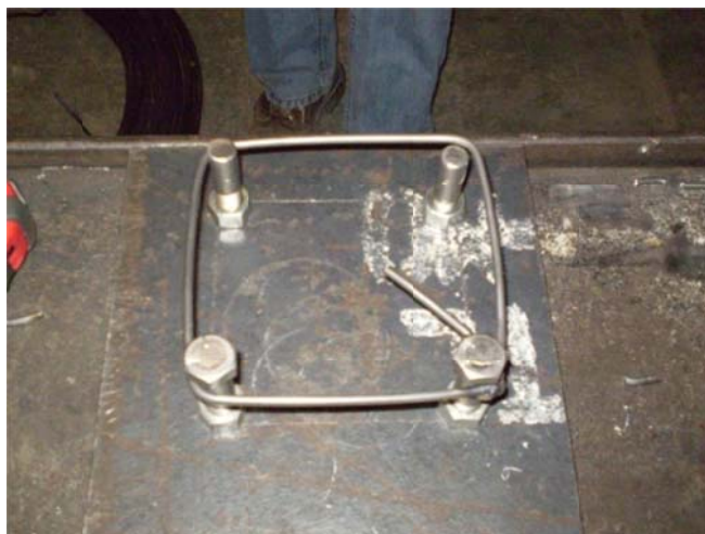
Figure 3.5.7: Bending of column stirrup
