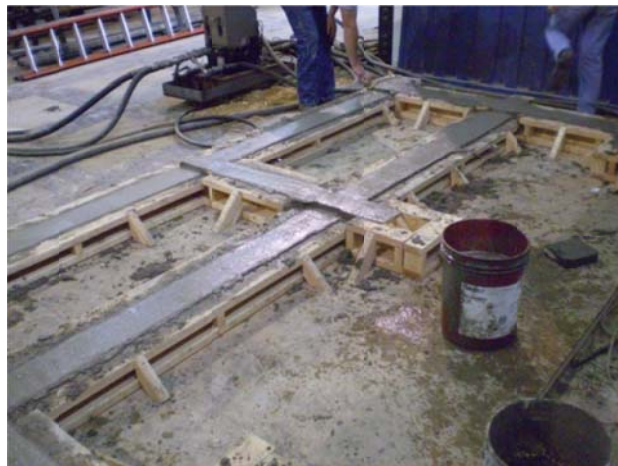
Figure 3.5.22: Poured concrete frame
