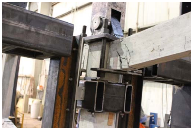
Figure 4.2.10: Crack forming near center column
