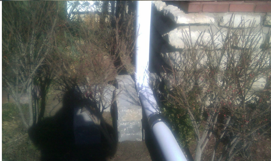
Figure 6. Winterized rain garden connection, looking north. 12/02/10
