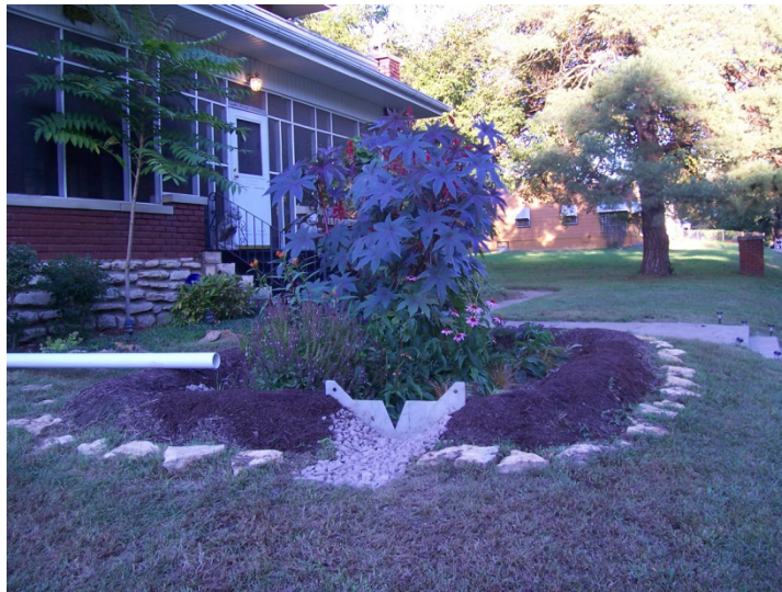
Figure 5.3 Weir outlet structure, shown at center.
