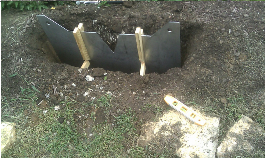
Figure 2. Weir installation. 09/23/10
