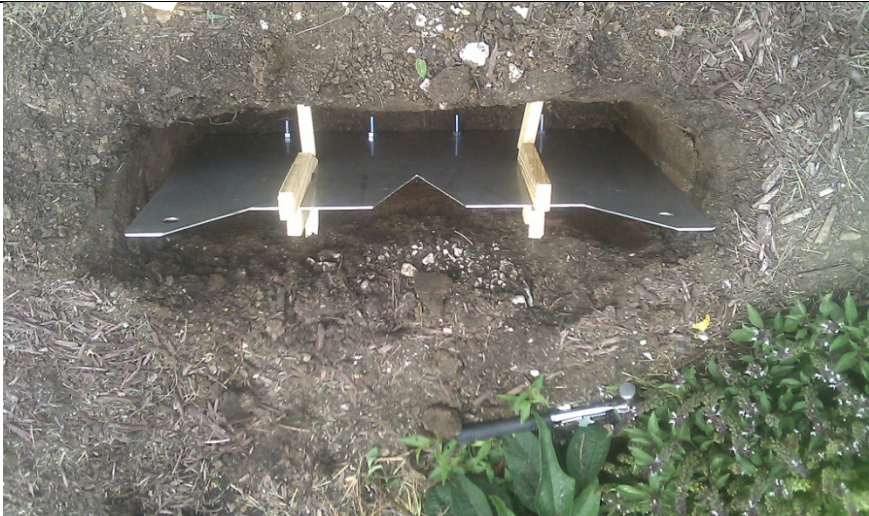
Figure 1. Weir installation. 09/23/10
