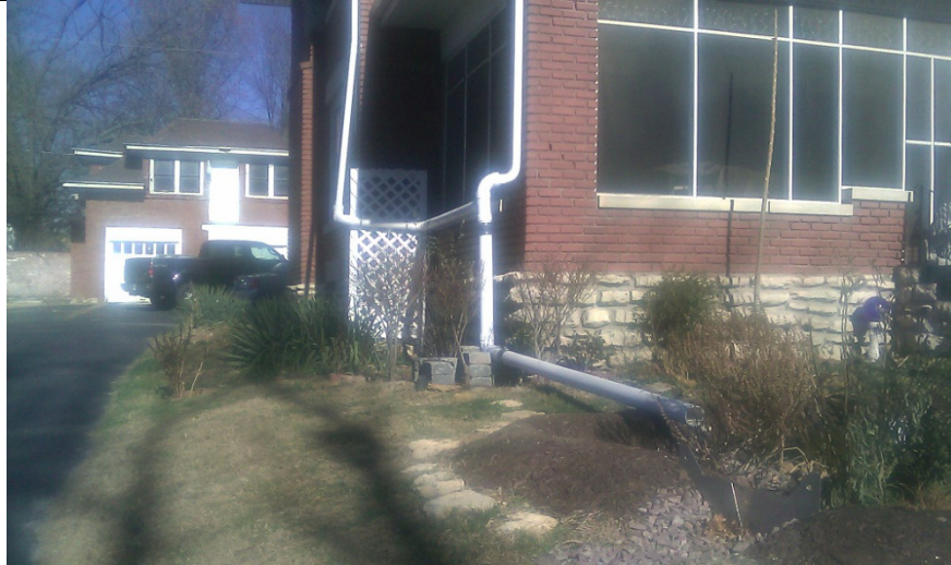
Figure 5. Winterized rain garden connection, looking north. 12/02/10
