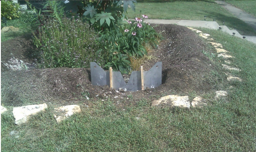
Figure 4. Weir installation. 09/23/10
