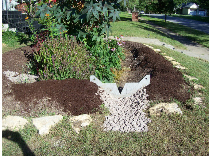
Figure 7.3 V-notch weir at rain garden outlet.
