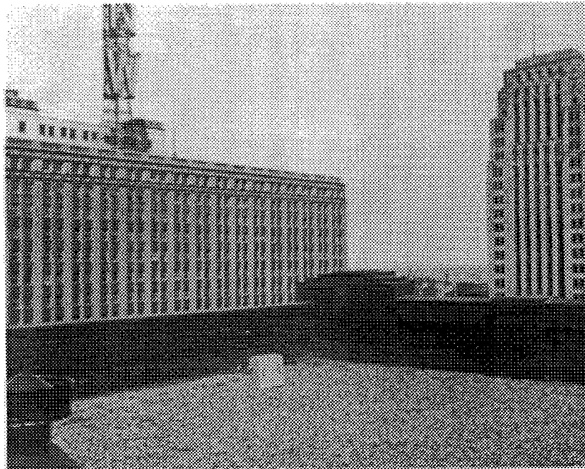
Fig. V-11 Typical roof top sampler location.
