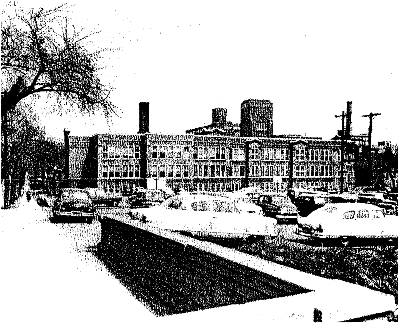
CLINTON SCHOOL, LOOKING NORTH FROM 29 th STREET
