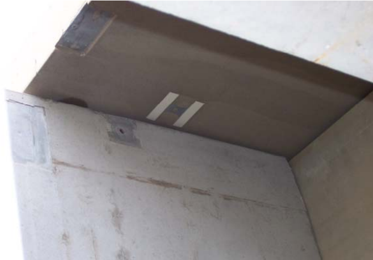
Figure 2: Improperly Located Embed Connection Plates
