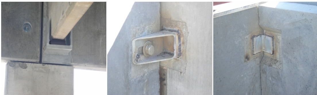
Figure 3: Common Precast Connections Subjected to Eccentric Shear
