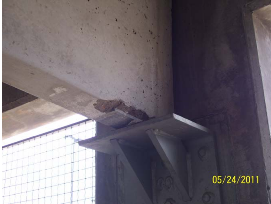
Figure 5: Post-Installed Corbel Assembly using an Adhesive Anchor System
