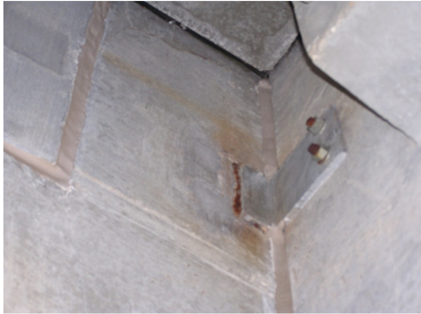
Figure 4: Common Precast Welded Repair using an Adhesive Anchor System
