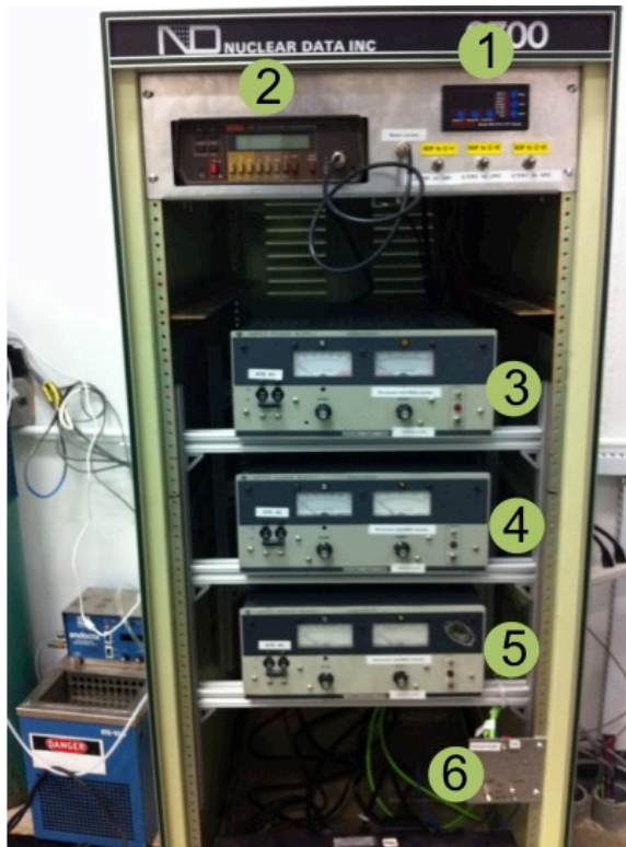
Figure 4.10 Electronics tower for the beamline
