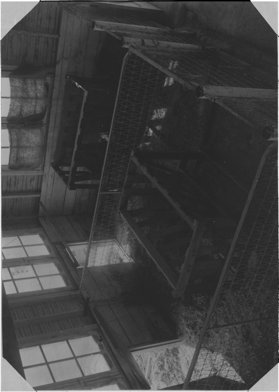
Fig. 4. Interior view of hog barn, showing Arrangement of feed racks and feed troughs.
