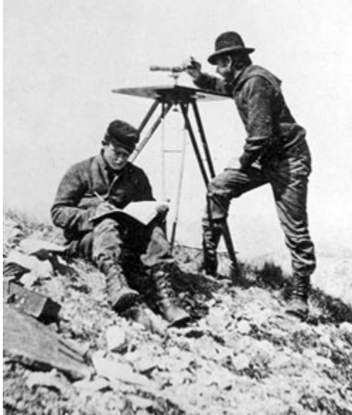
Figure 1.1 Plane-table surveying by USGS topographers (source: [5])
