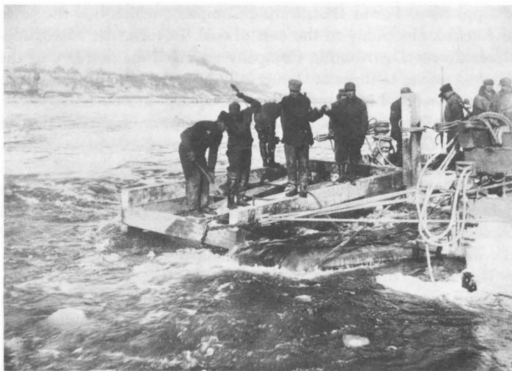
Building the cofferdam for the Keokuk dam, 2 January 1912.
