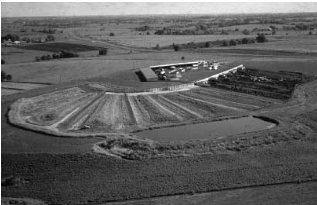
Figure 4. Lot runoff from this beef feeding facility is routed to a lagoon for later land application by irrigation.
