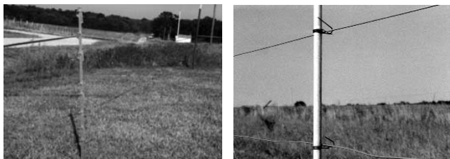
Figure 6. These posts do not require insulators. (Left) Plastic fence post with molded-on wire/tape clips. (Right) Fiberglass rod with wire clips.
