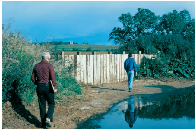
Figure 10. This picket dam drains directly into a holding pond below the storage structure.
