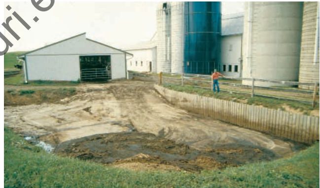
Figure 1. Picket dams provide storage for manure while allowing water to drain away.
