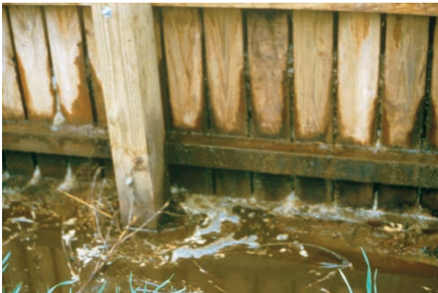
Figure 9. This picket dam drains through ¾-inch openings between vertical 2-inch x 6-inch treated wood pickets.
