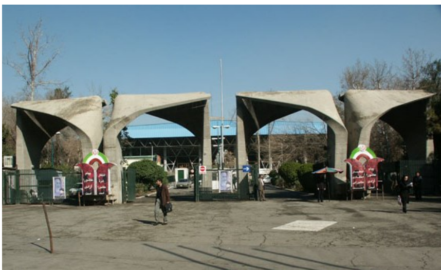
Figure 4-7: Tehran University's campus (1934) (source: Tehran University website)
