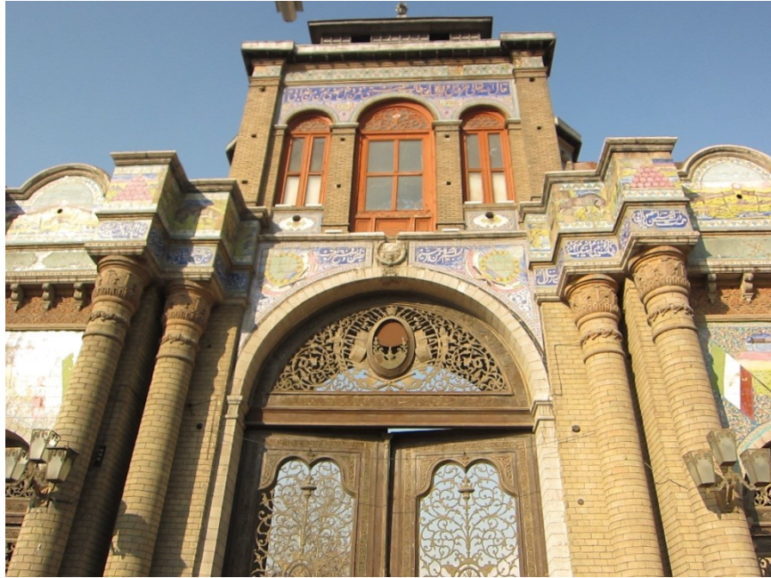
Figure 4-5: The entry gateways of Meidan Mashgh (1931, today's Bagh-e-Melli)
