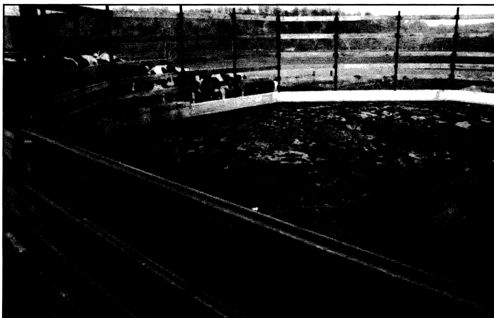
A full concrete manure storage tank with the surface covered with floating bedding. The fence prevents accidental entry into the tank.
