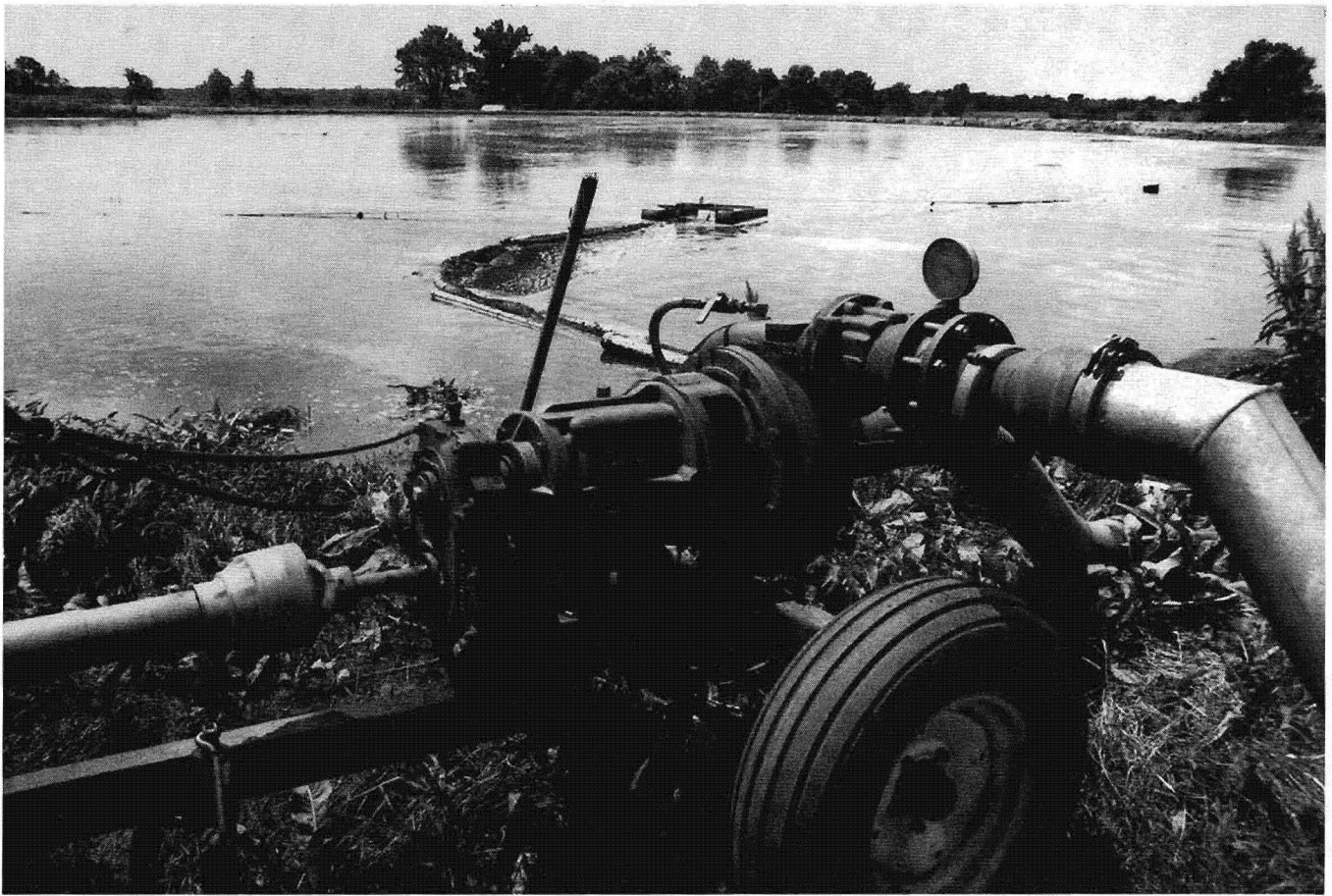
Figure 8. This booster pump is fed by a chopper pump submerged in the lagoon.
