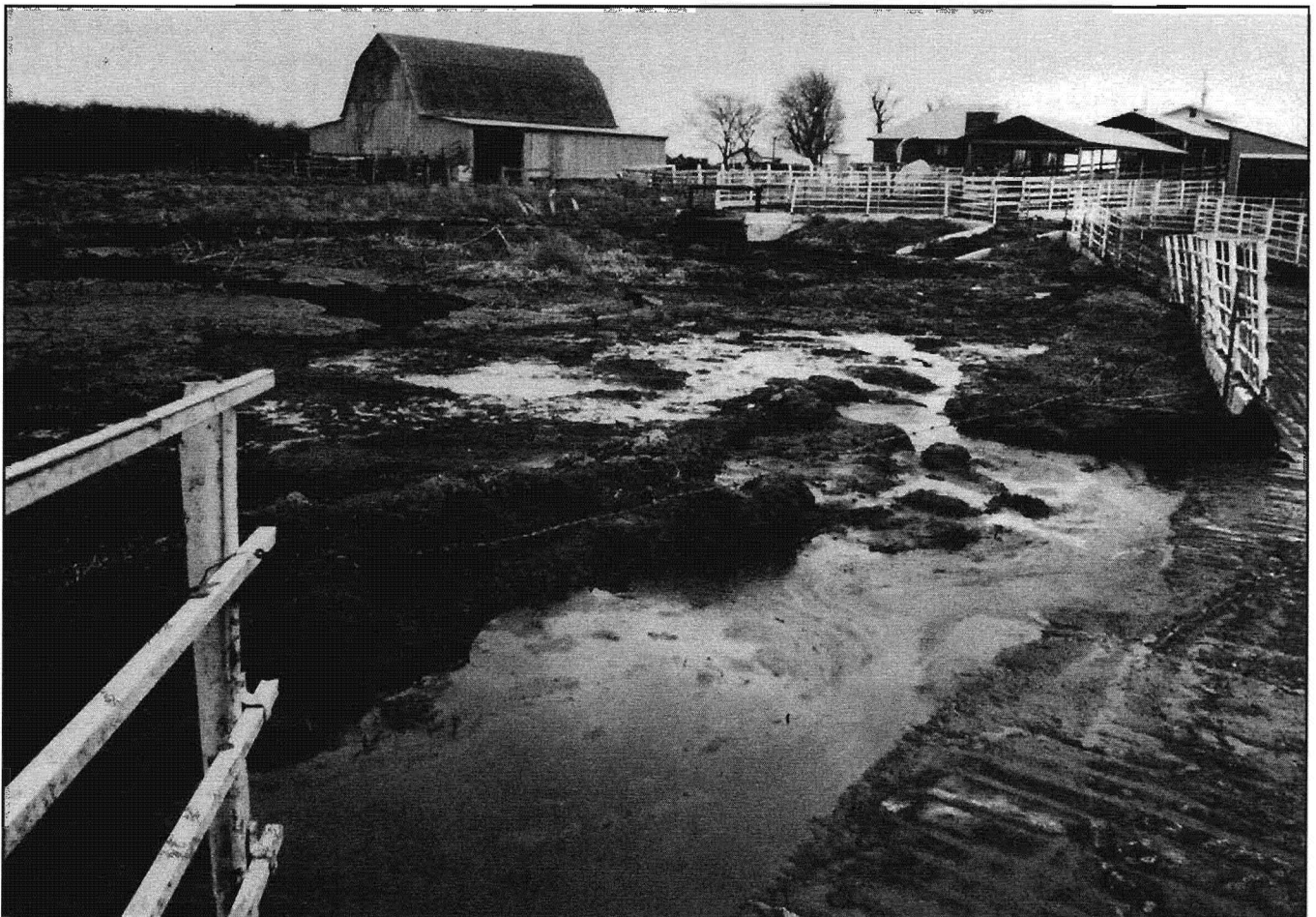
Crusted and settled solids have significantly reduced liquid volume in this dairy lagoon.
