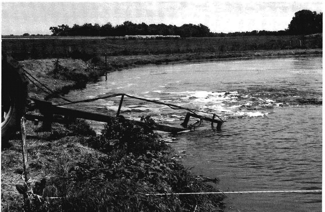
Figure 13. Placing the agitator at an angle creates a swirl effect in the lagoon.
