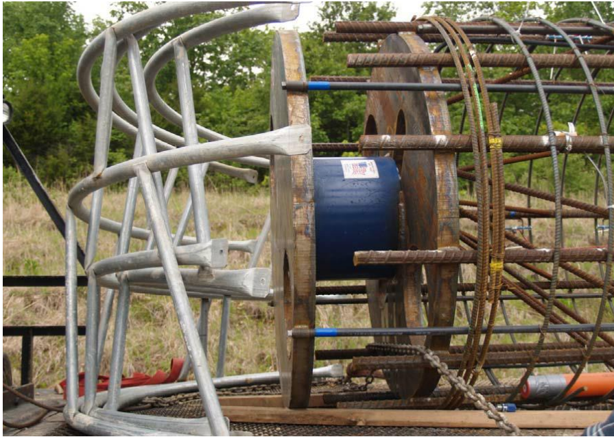
Figure 5.11. O-Cell® welded to top and bottom plates at the end of a rebar cage.
