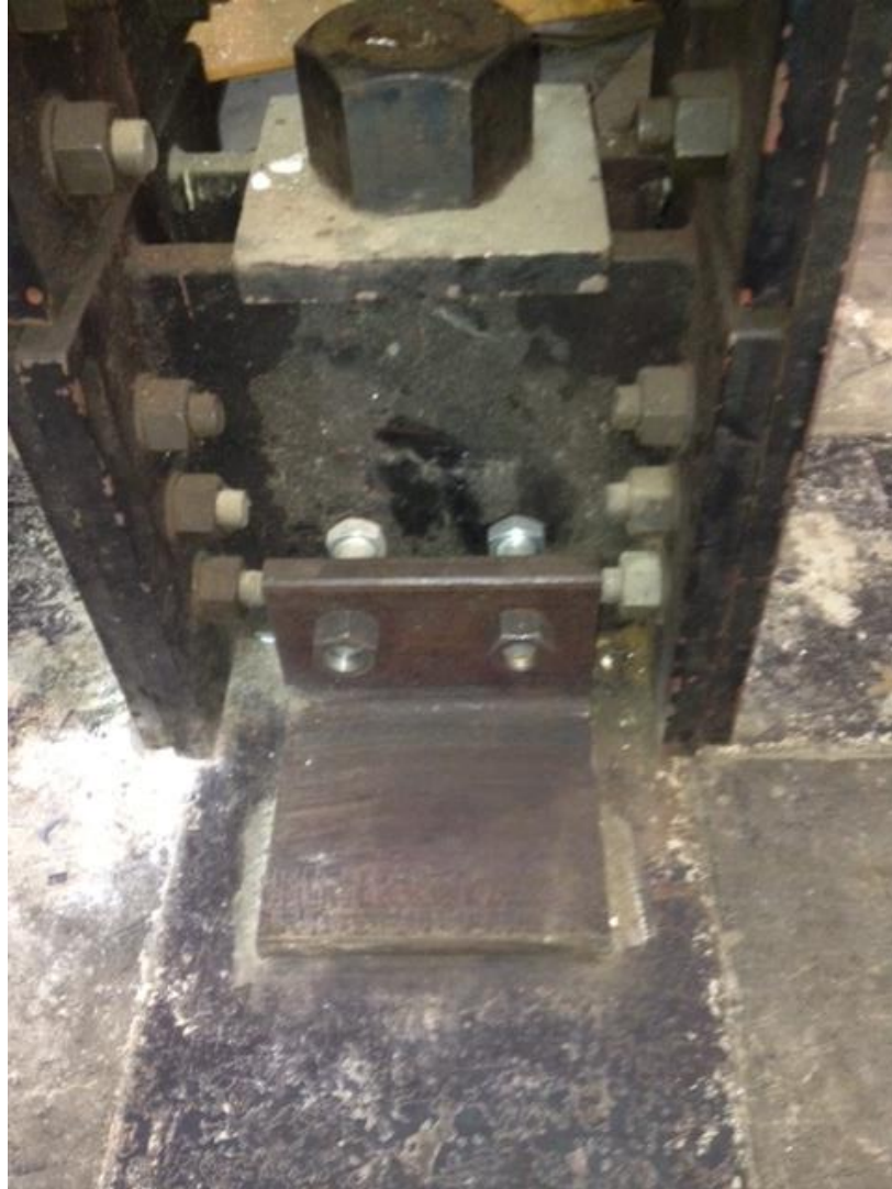
Figure 3.4.5 – Added bracing to prevent the support columns from sliding during restrained testing.
