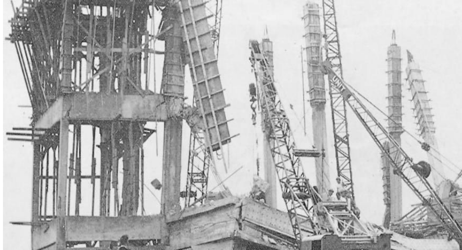
Figure 2.3.1 – Photo of collapsed structure in Jackson, Michigan (Aberdeen Group 1956).
