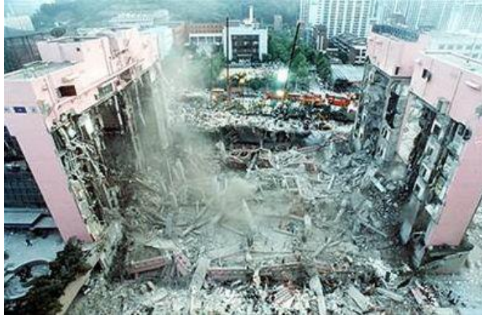
Figure 2.3.3 – Photo of the collapsed Sampoong Department Store Building (Gardner et al 2002).
