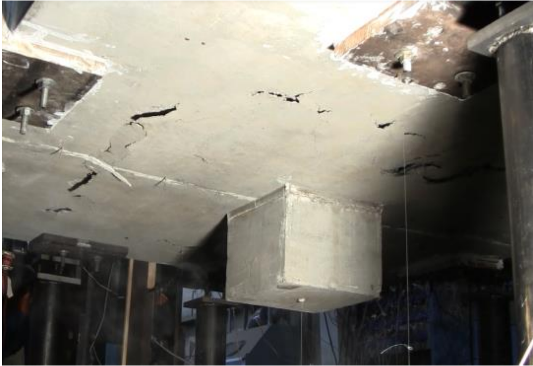
Figure 4.2.3.12 – Underside of the 1.0% restrained slab just after the punching failure occurred.
