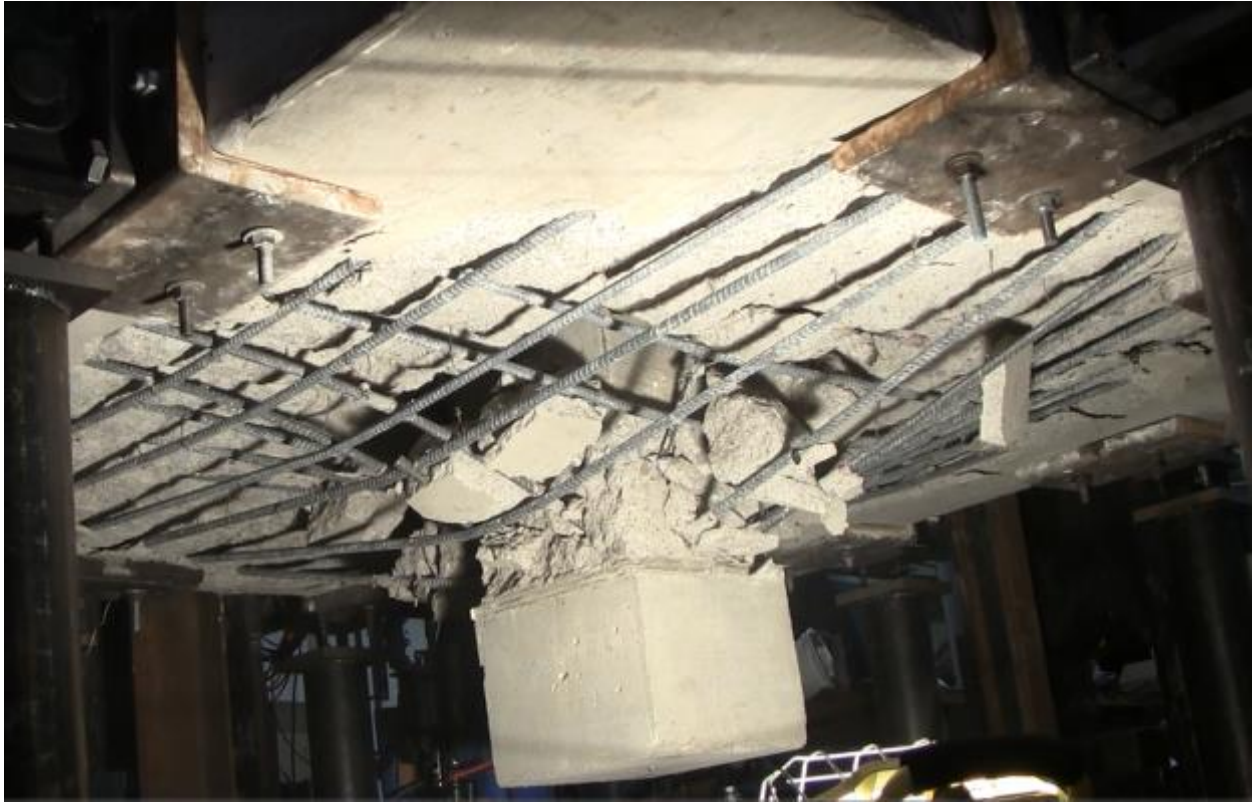
Figure 4.1.4.2 – Underside of the 1.0% unrestrained slab at the conclusion of the testing.
