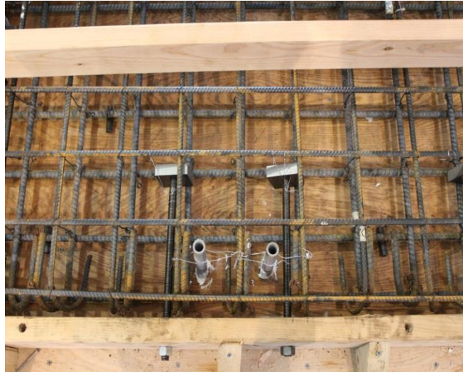
Figure 3.4.4 – Anchorage area prior to casting slab.
