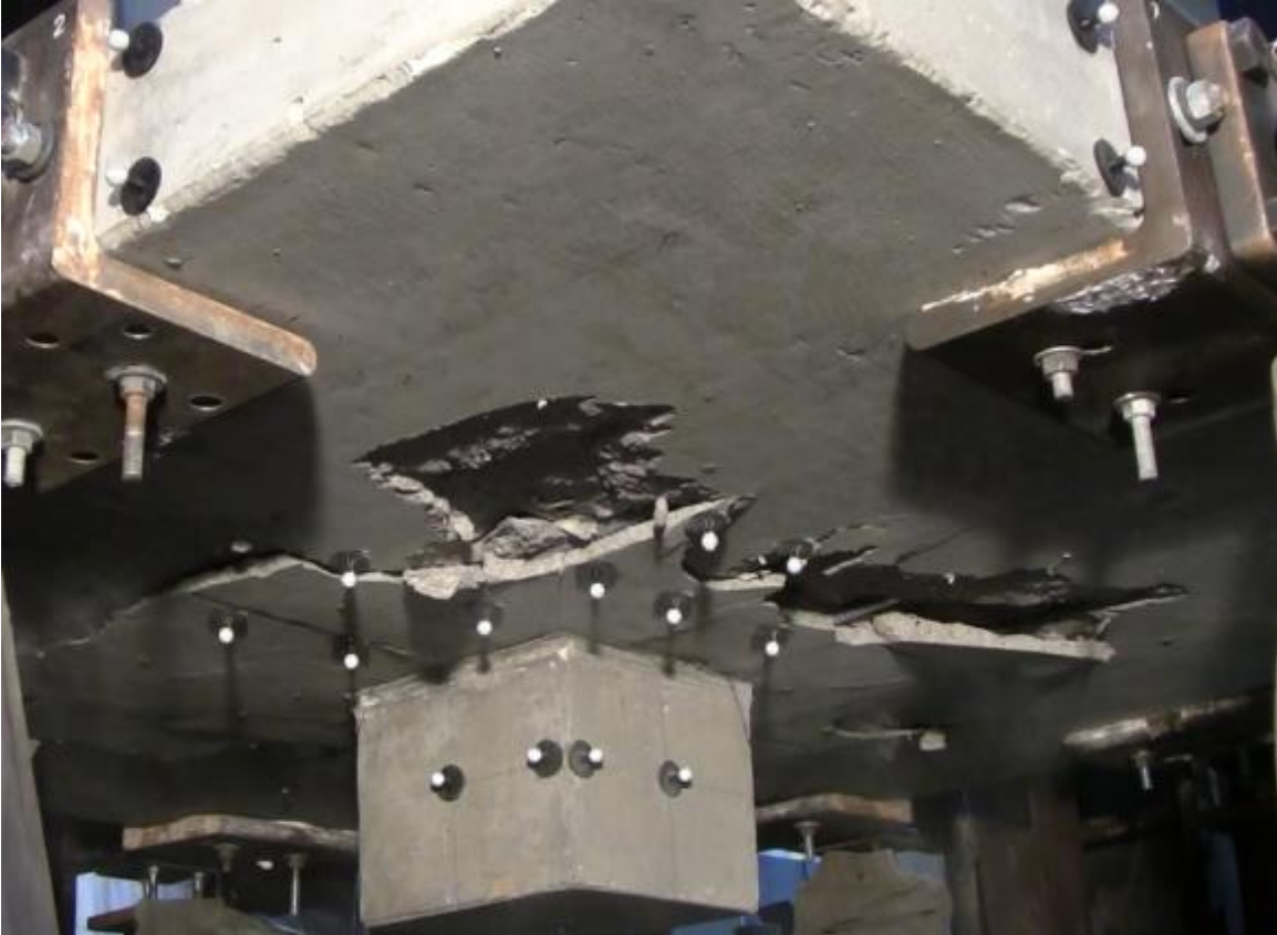
Figure 4.2.1.12 – Underside of the 0.5% restrained slab just after the punching failure. The slab bottom was instrumented with markers to record displacements via video.
