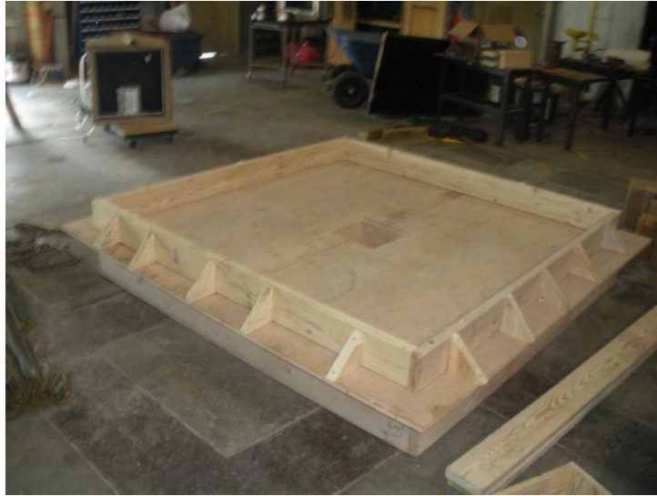
Figure 3.3.1 – Formwork for the slab specimens without top column stub formwork in place.
