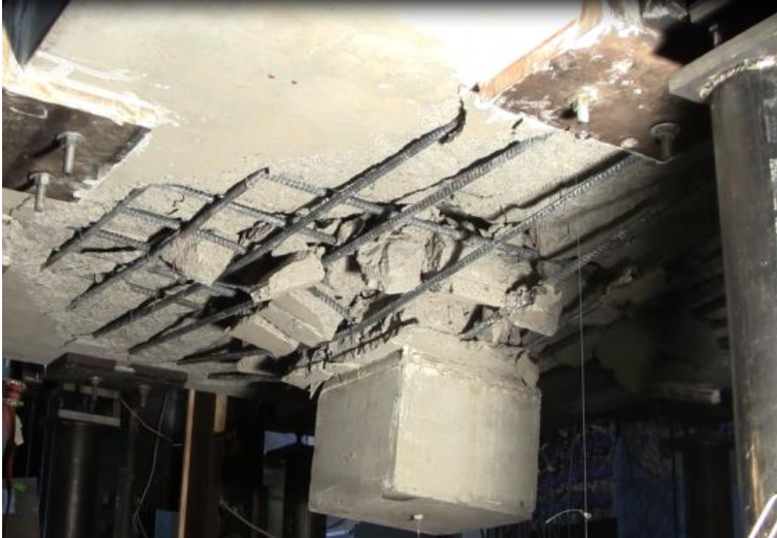
Figure 4.2.4.2 – Underside of the 1.0% restrained slab at the conclusion of the testing.
