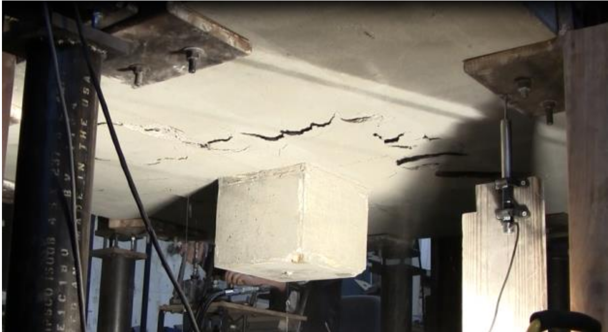
Figure 4.1.1.2 – Underside of the 0.5% unrestrained slab just after the punching failure.
