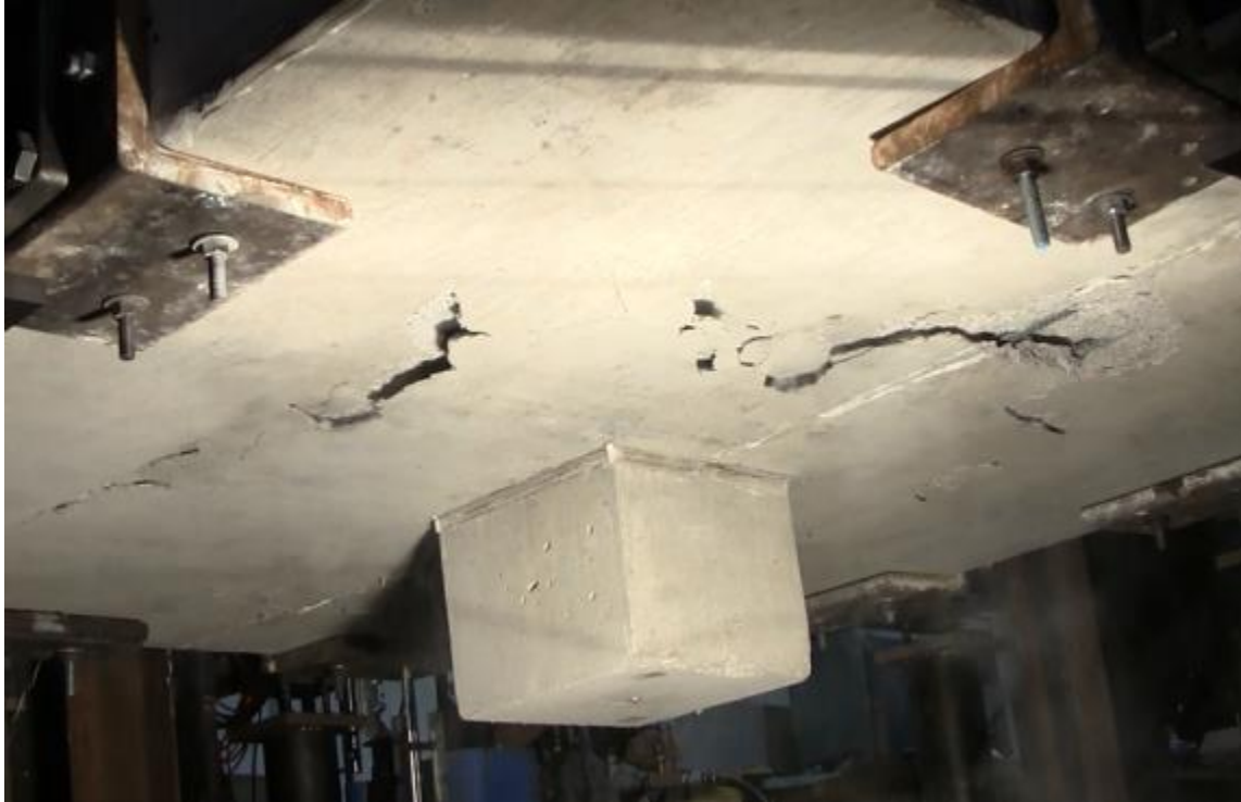
Figure 4.1.3.9 – Underside of the 1.0% unrestrained slab just after the punching failure.
