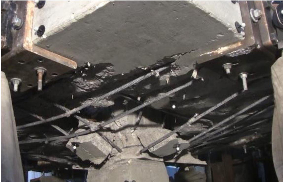
Figure 4.2.2.2 – Underside of the 0.5% restrained slab at the conclusion of the testing.
