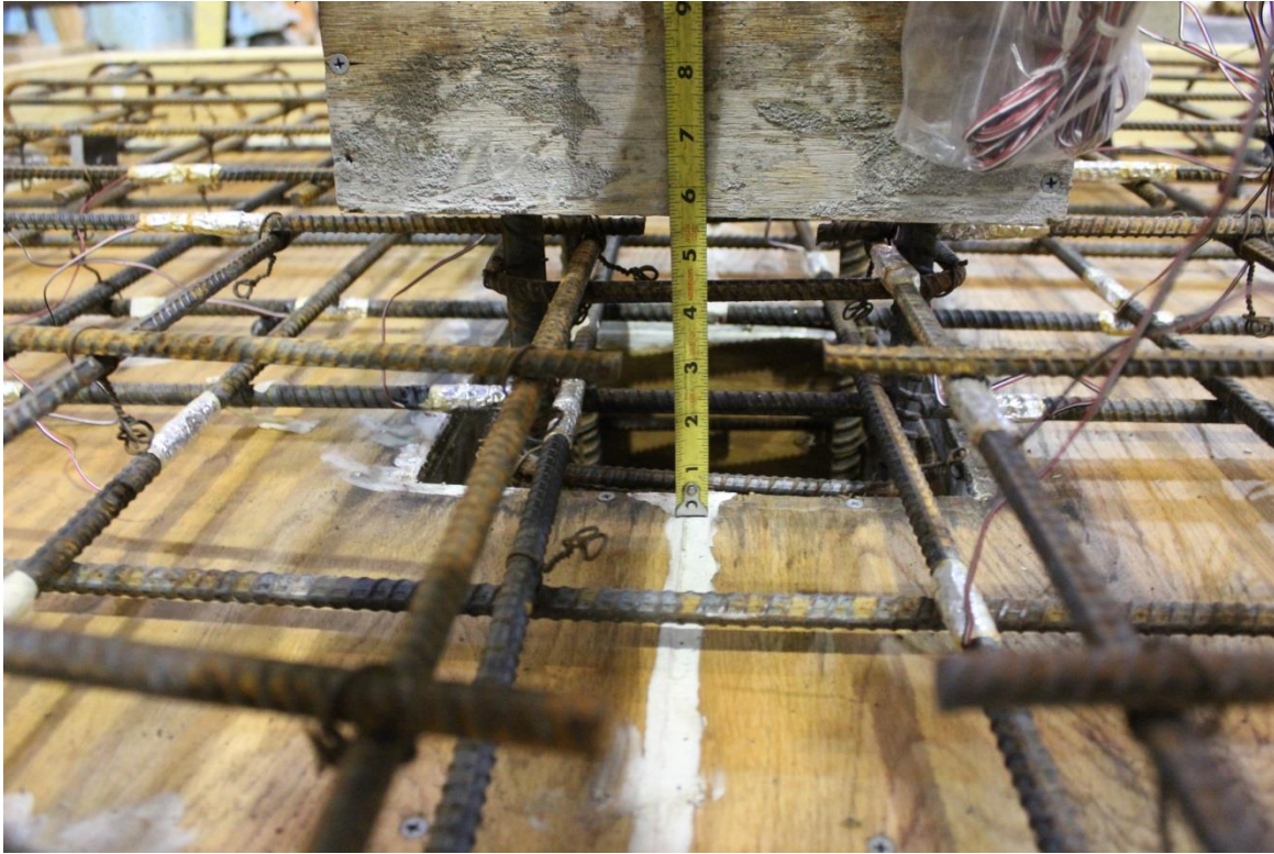
Figure 3.3.2 – Picture of slab formwork showing slab depth and reinforcement depths.
