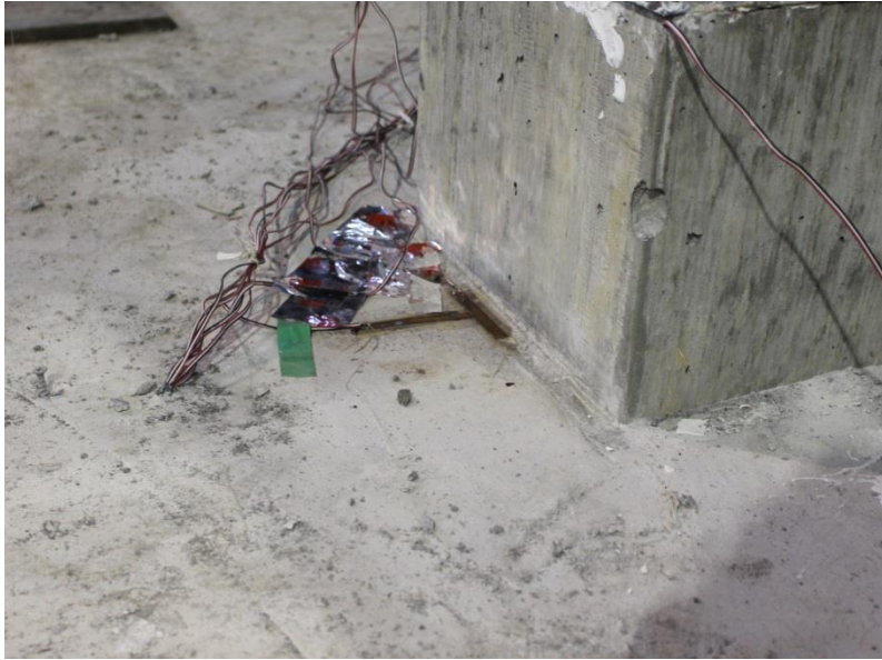
Figure 3.5.5 – Picture of concrete gages in position on the slab against the face of the column.
