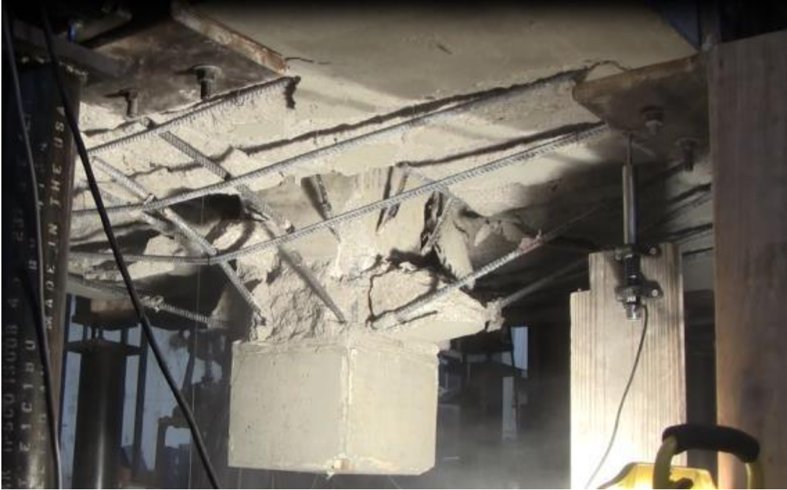
Figure 4.1.2.3 – Underside of the 0.5% unrestrained slab at the conclusion of the test.
